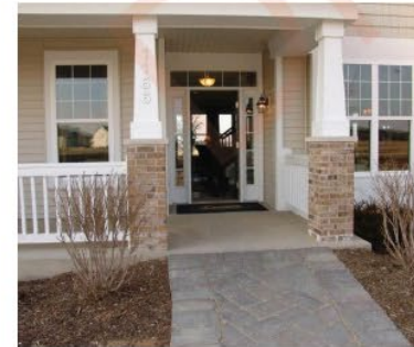
Figure 54. Gently sloping ramps can provide no-step access to grade-related homes.
