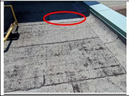
**Photo 3**: Degranulation (darker areas) of the membrane which is indicative of the age. Will accelerate UV deterioration of the membrane. Previous patch repairs (lighter coloured membrane patch).
