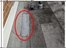
Photo 6: Previous patch repairs.
