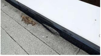
**Photo 4**: Blister at the roof perimeter. Note with increase in temperature blisters become larger this increases the thermal expansion/contraction of the membrane. This will increases wear on the membrane (e.g. degranulation, cracking).
