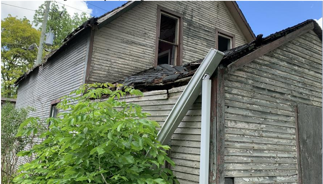
Rear tail of building – roof collapse. Main roof with hole (Heritage Section Photo)
