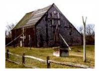
Buildings seriously damaged by storms or deterioration may need to be braced before architectural evaluations can be made. Photo: John Milner Architects. Photo: NPS
