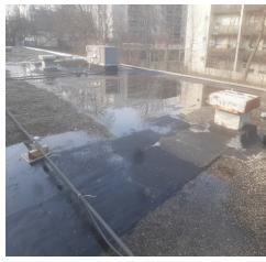
Significant ponding, numerous roof leaks throughout facility, patching attempts have not been successful.
