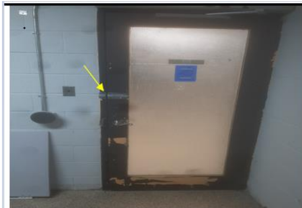
Photograph No. 9A – Accessible washroom door improper locking device.
