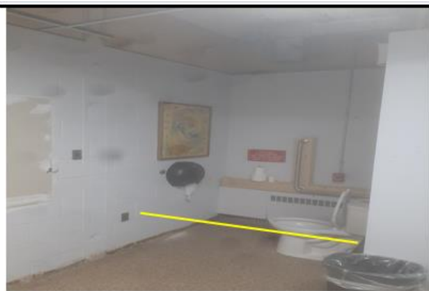
Photograph No. 9B – Accessible washroom has no partition.
