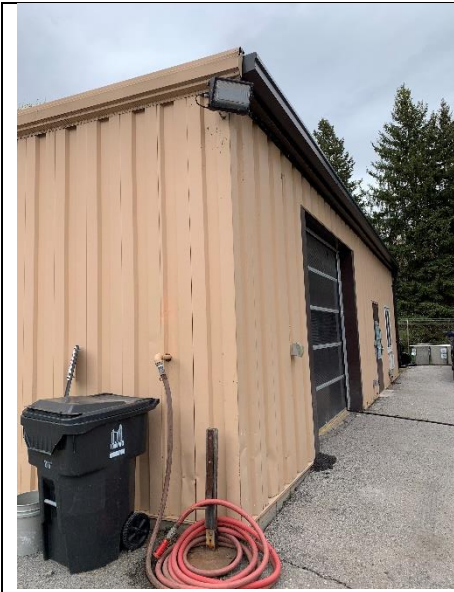
Shop - Metal Siding Repairs
