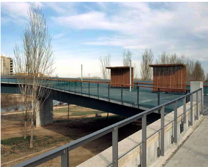
Figure 36: Segre River Active Transportation Bridge, Spain
