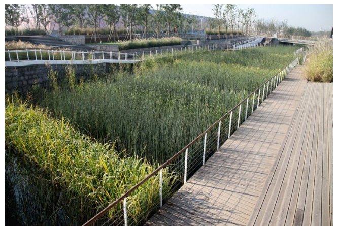
Figure 53: Ecological Flood Control, Houtan Park, Shanghai
