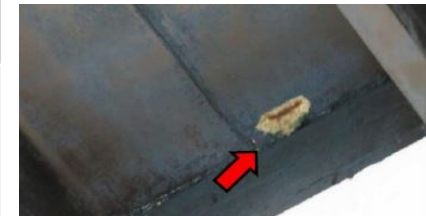
Image 2 – Concrete spall at underside of precast double-tee above swimming pool area
