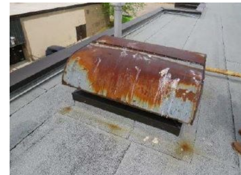
Image 4 – Existing HVAC infrastructure with galvanized coating corroded
