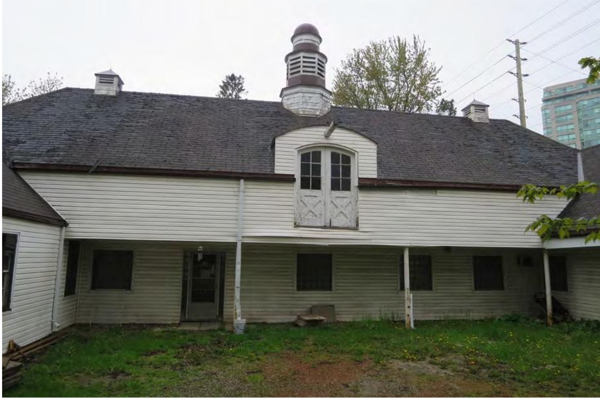
Stable Building (unoccupied)
