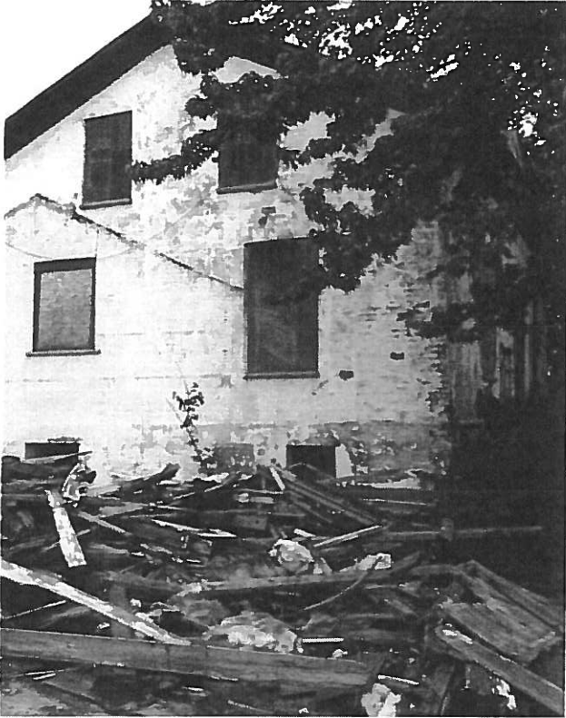
- South Elevation. Remnants of an existing addition.
