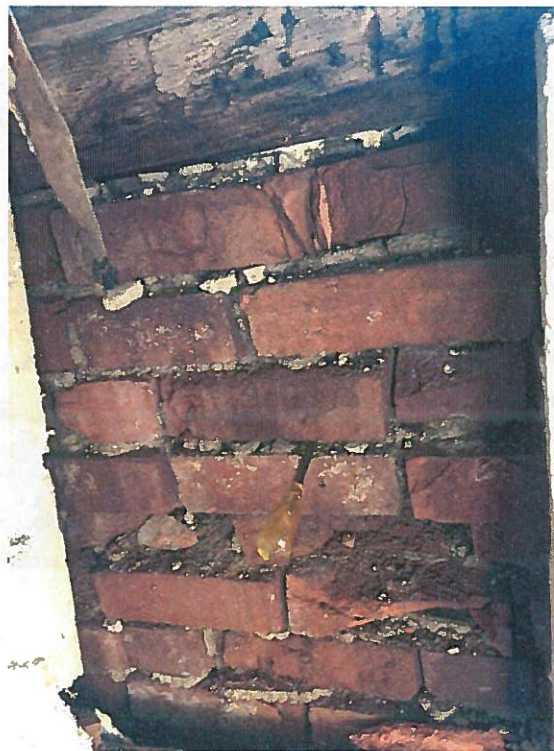
Wall at dormer location
