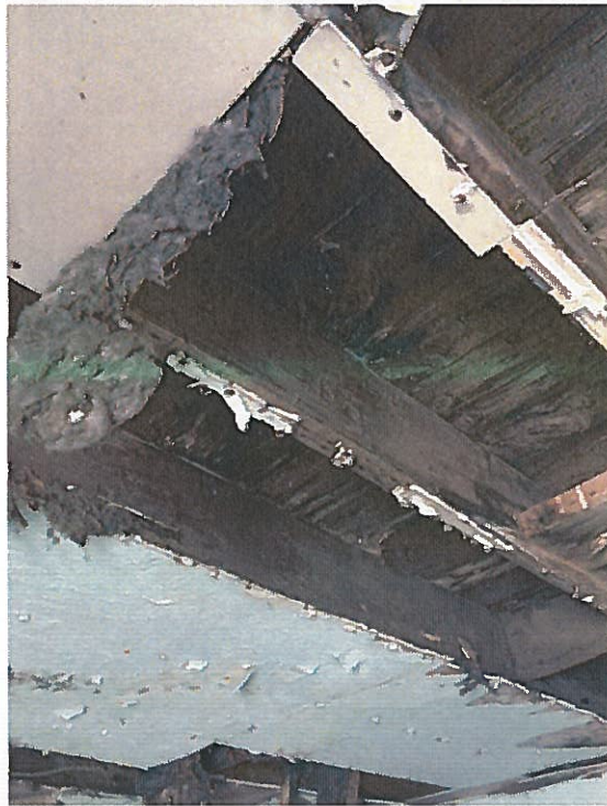
Roof joists at low roof
