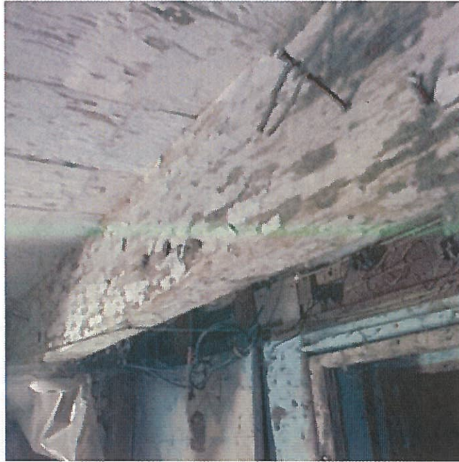
Main wood beam in basement
