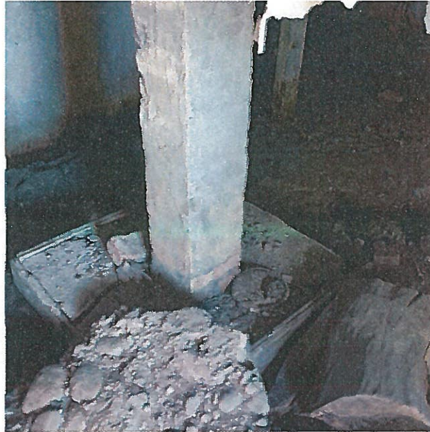
Brick pier under the beam in basement
