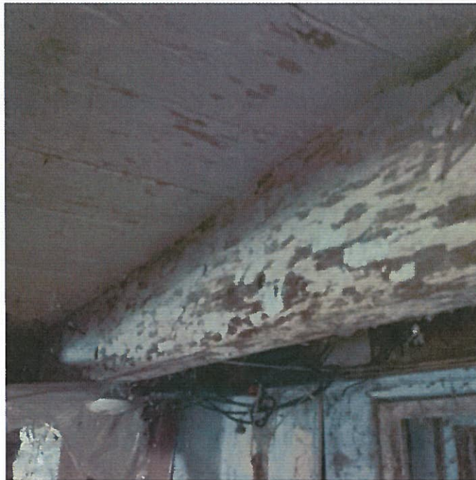
Main wood beam in basement
