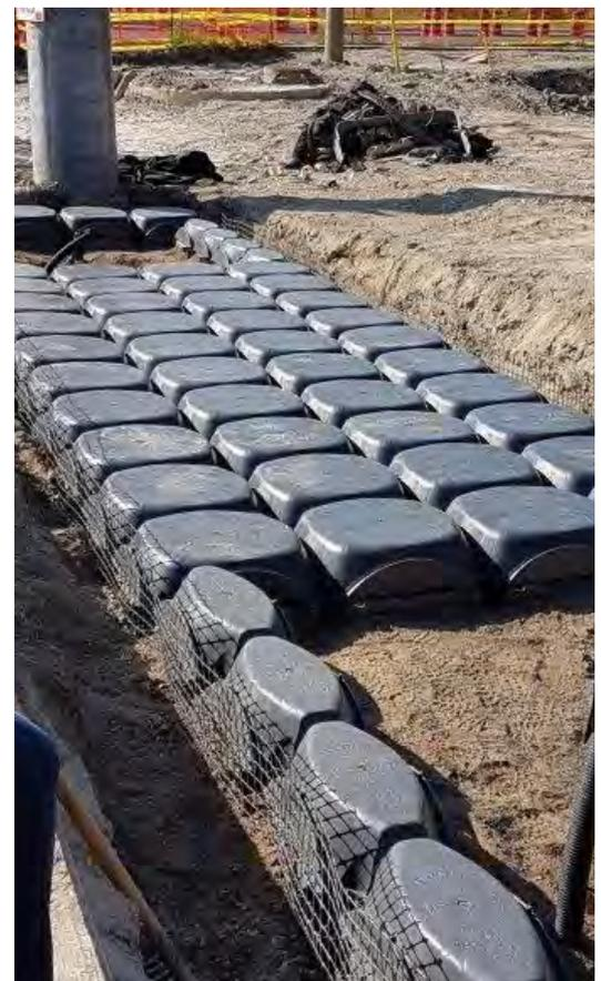
Installation of a soil cell system
