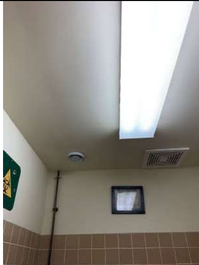
Washroom ceiling drywall
