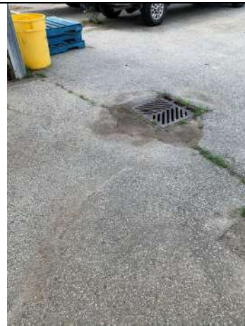
Central greenhouse asphalt
