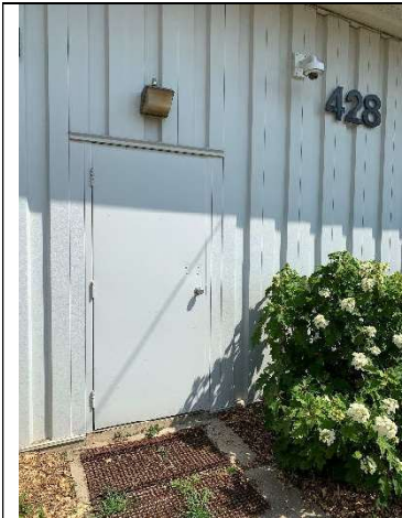
Painted metal door with frame
