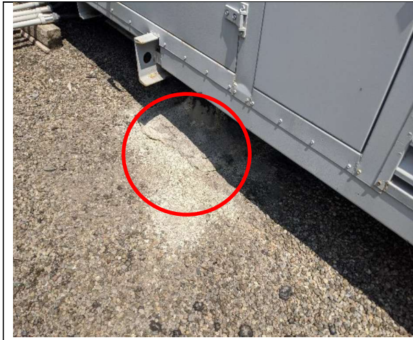
Photo 1: Roof repair to address leak.
