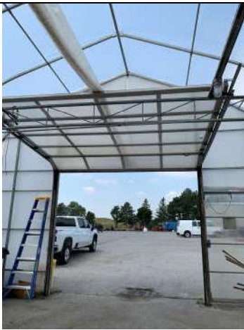
Central greenhouse overhead door
