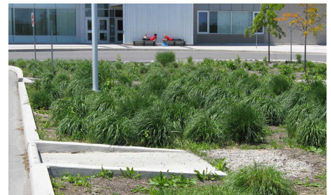
Image 7.35-7.37 Low-Impact Development practices at Markham's Bill Crothers Secondary School include bioretention areas, vegetated swales, constructed wetland type stormwater management facilities, and a rainwater harvesting system. Many streets within Markham Centre have good tree canopies.
