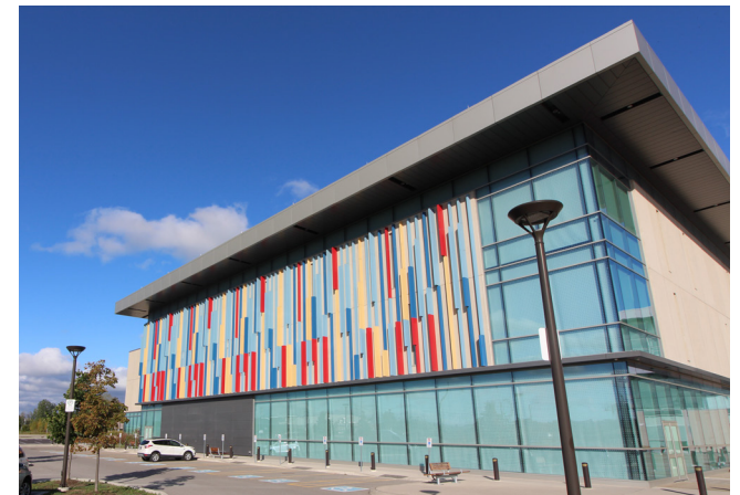
Image 2.2, 2.3 Major public investments like the Viva Rapidway and Pan Am Centre contribute to Markham Centre's transformation.
