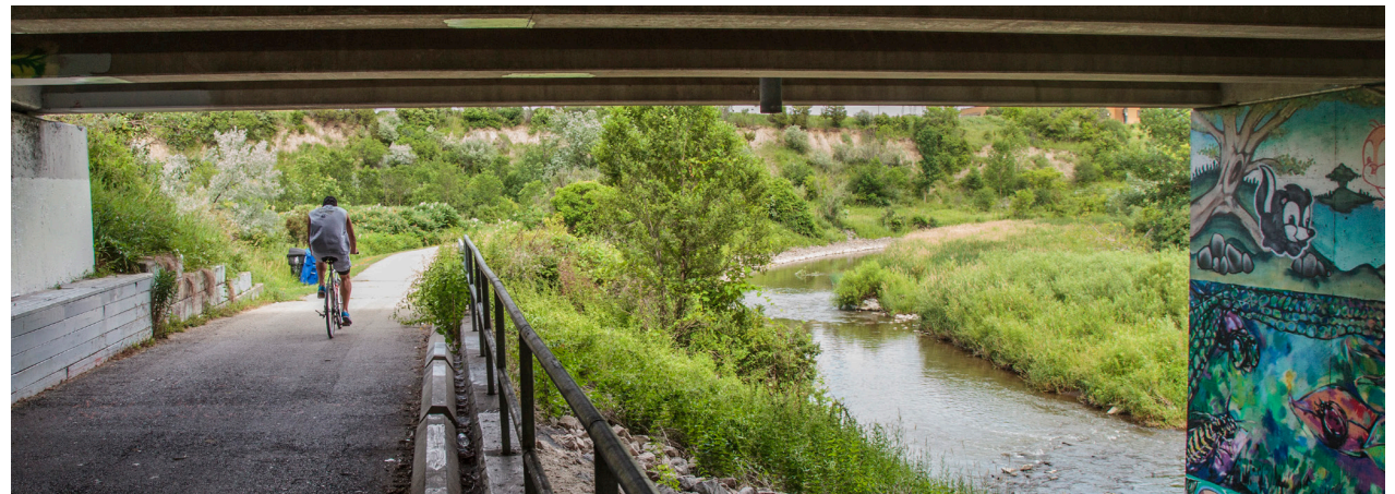
Image 7.33, 7.34 The Humber River Valley in western Toronto contains trails of varying intensity, connecting neighbourhoods and linking together parks along an open space system.
