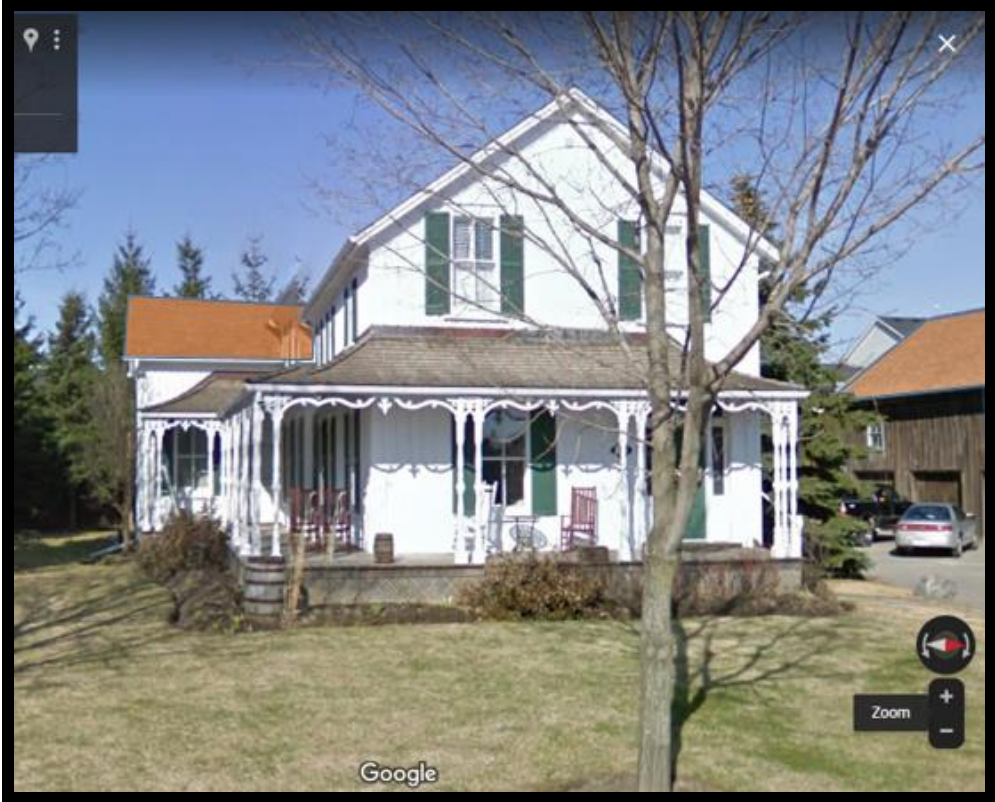
Google Street View Image from 2009 showing visibility of proposed metal roofs in orange colour
