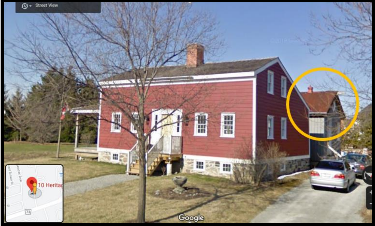
Home at 10 Heritage Corners Lane with salvaged galvanized roofing on new addition
