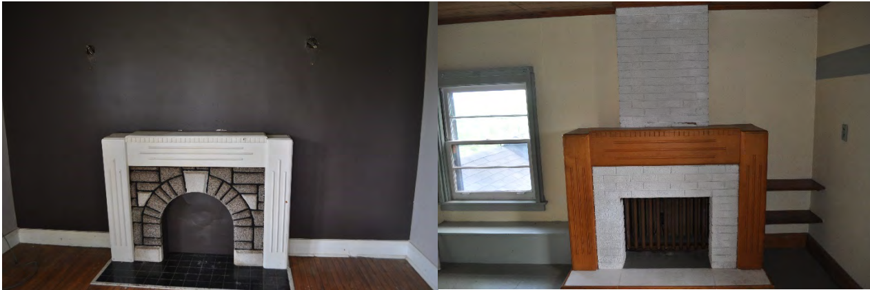
Photo 8: Fireplaces, first floor (left), second floor (right)
