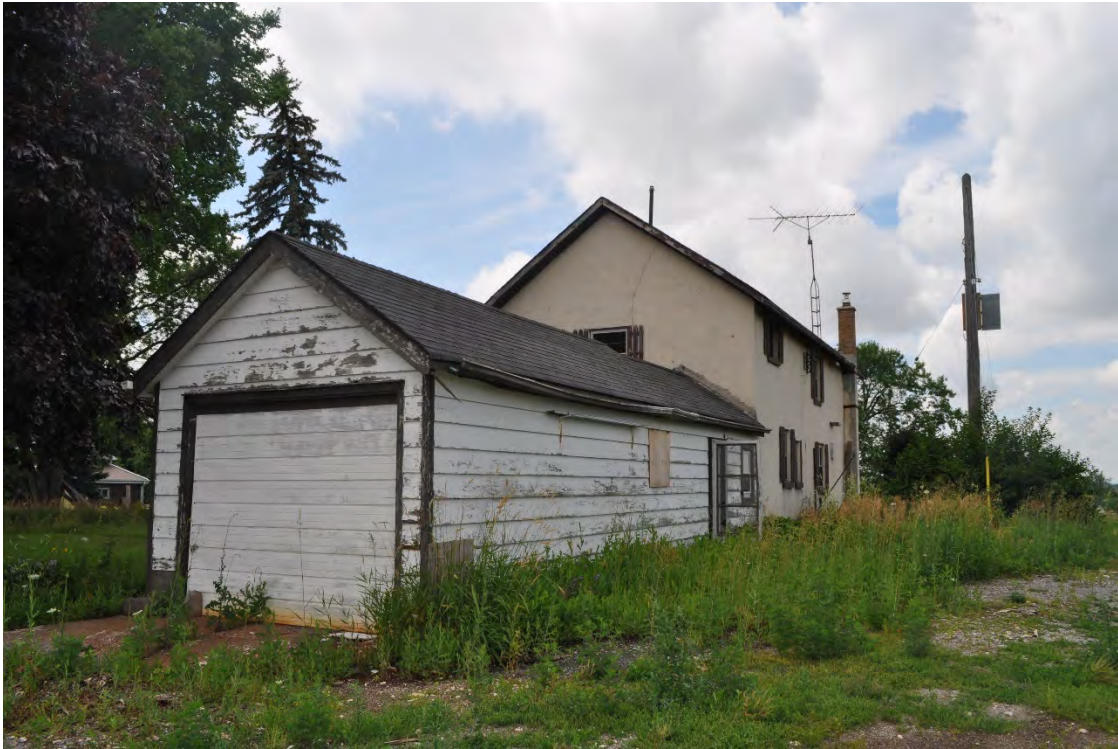
Photo 4: 4638 Major Mackenzie Drive East, east and north (rear) elevations
