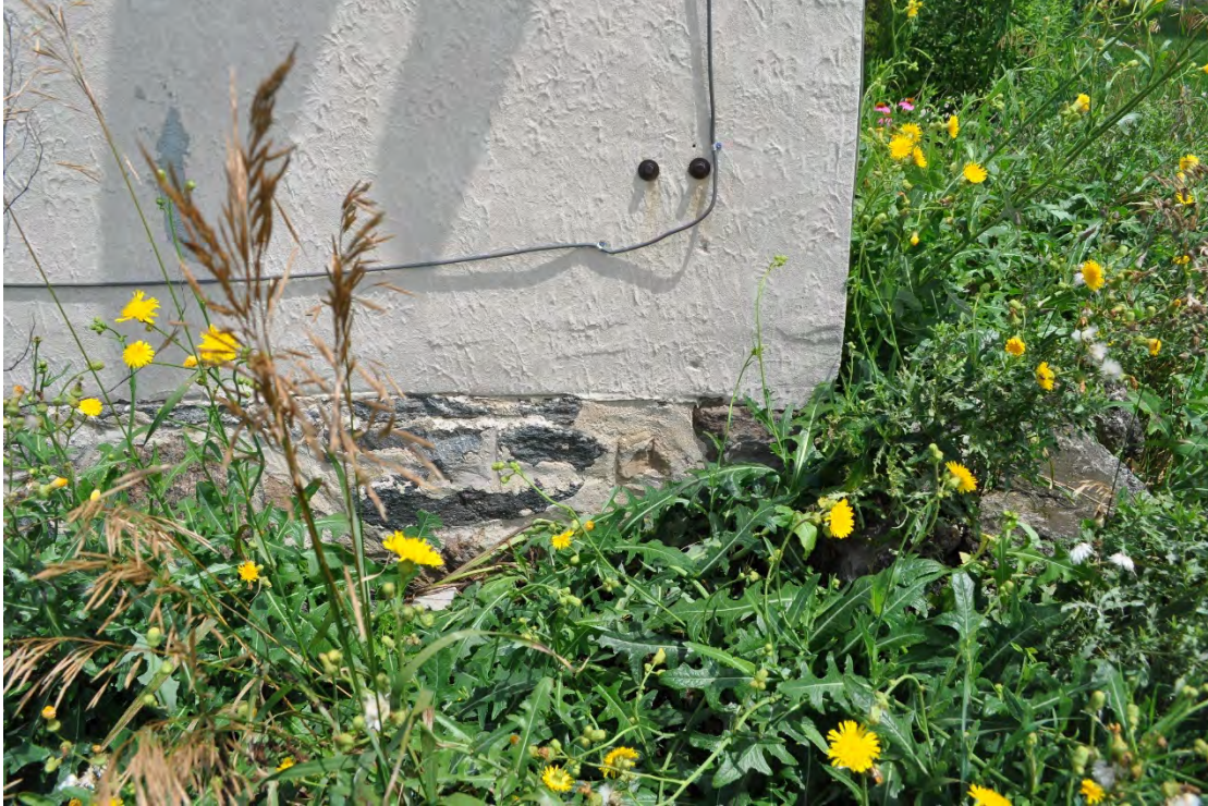
Photo 6: Detail of foundation stones along west elevation
