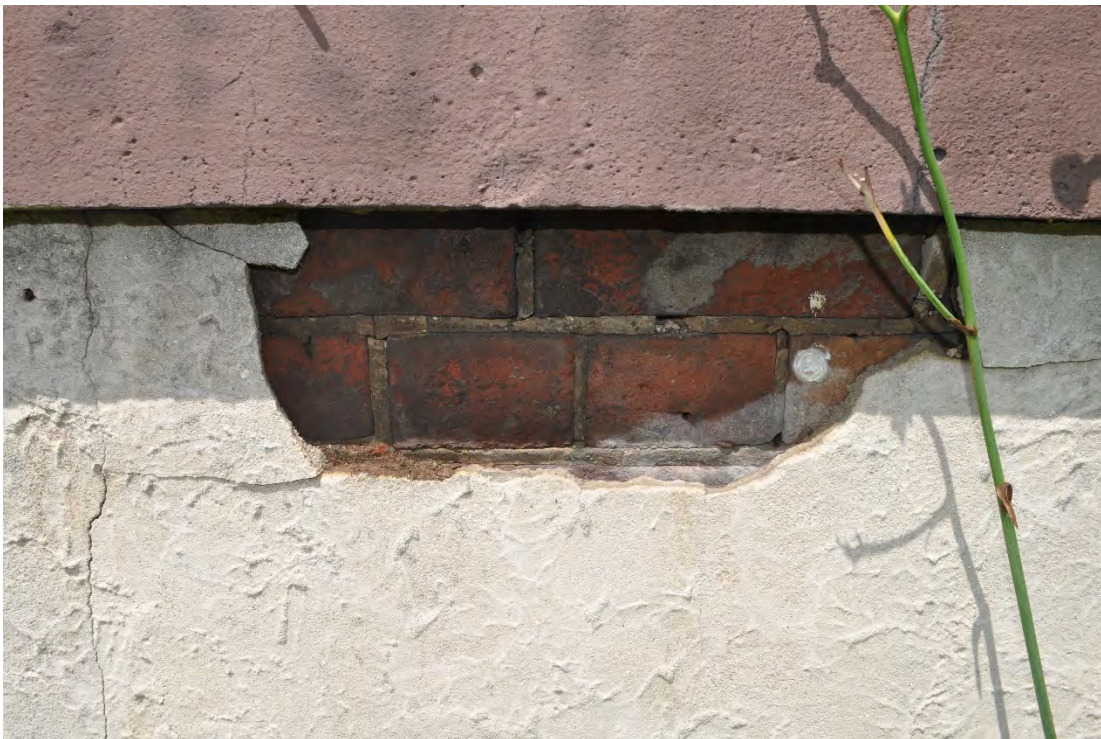
Photo 7: Detail of foundations, near southeast corner of structure
