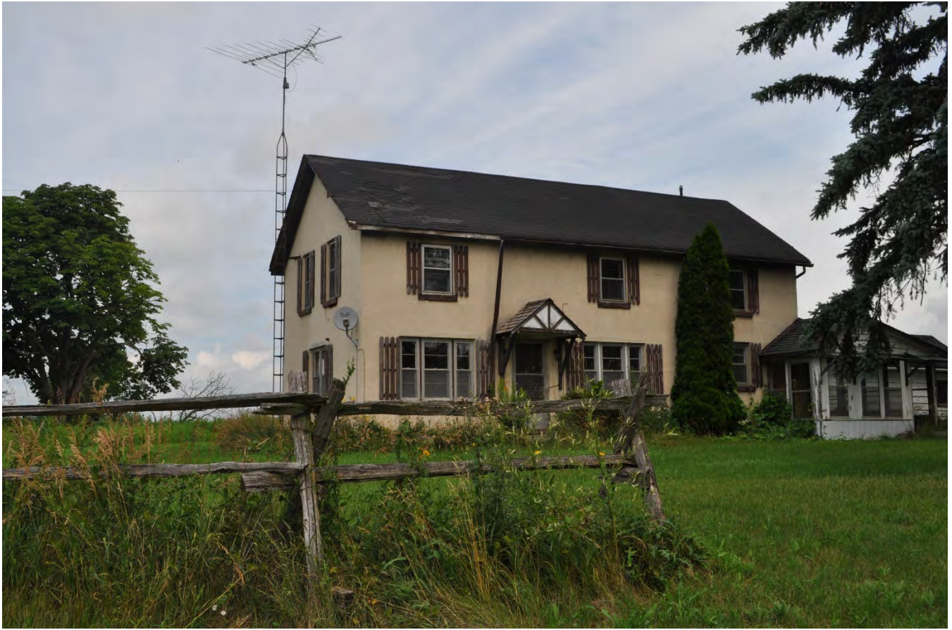
Photo 1: 4638 Major Mackenzie Drive East, front elevation facing north
