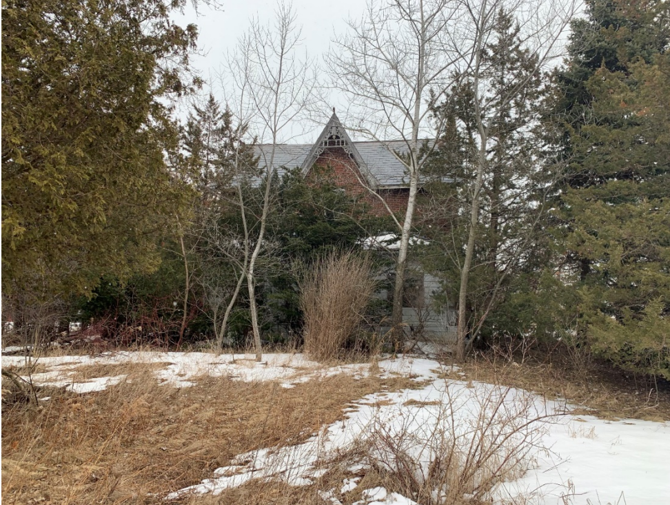
Figure 14: View front façade (CU 2020).
