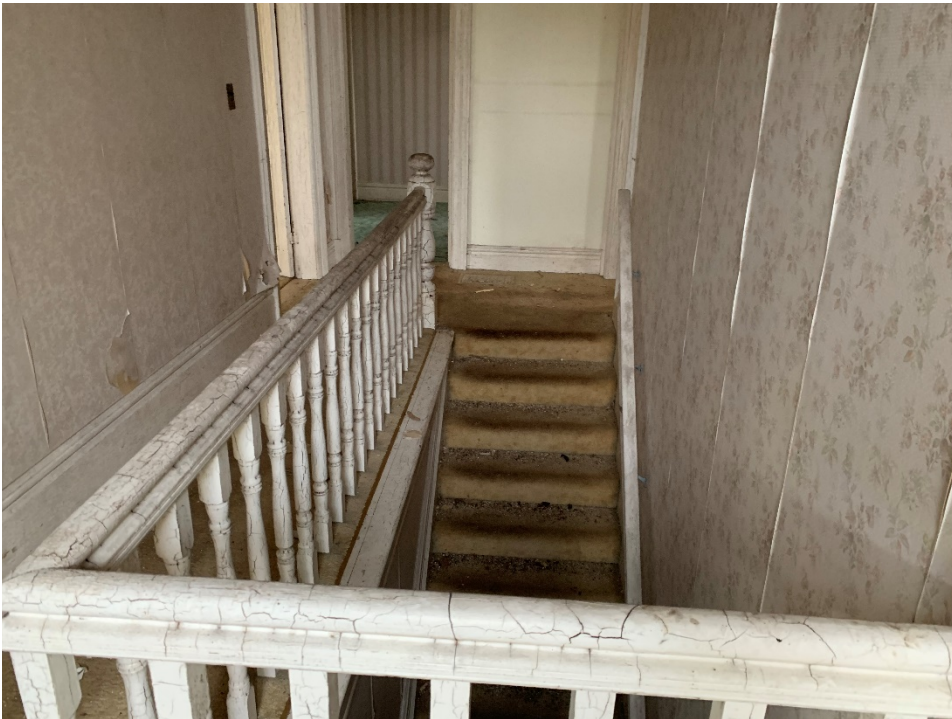
Figure 21: Detail of wooden staircase (CU 2020).
