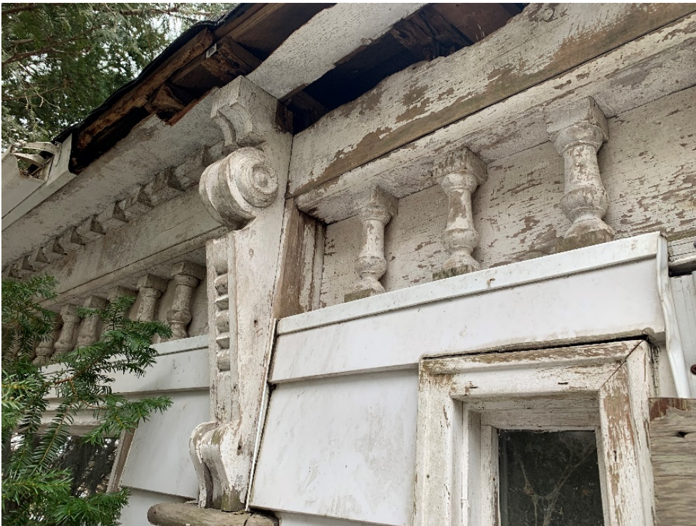
Figure 17: Detail of woodwork along north porch (CU 2020).
