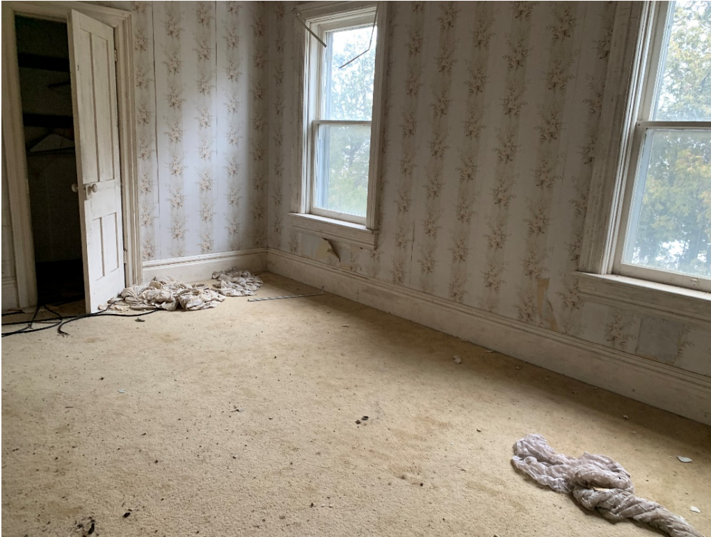
Figure 22: Typical view of upper floor room (CU 2020).
