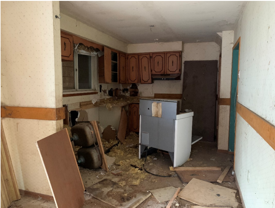
Figure 19: Interior, two-storey addition (CU 2020).
