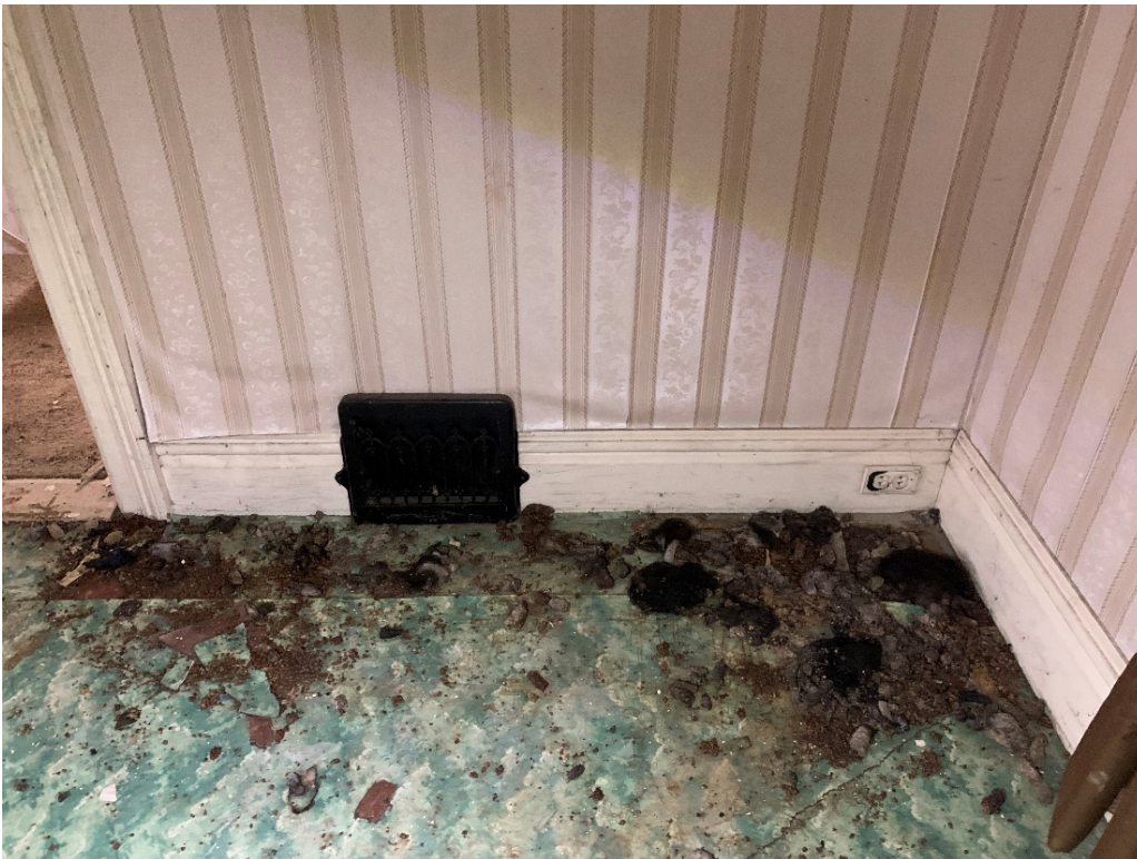
Figure 23: Metal ventilation grate (CU 2020).
