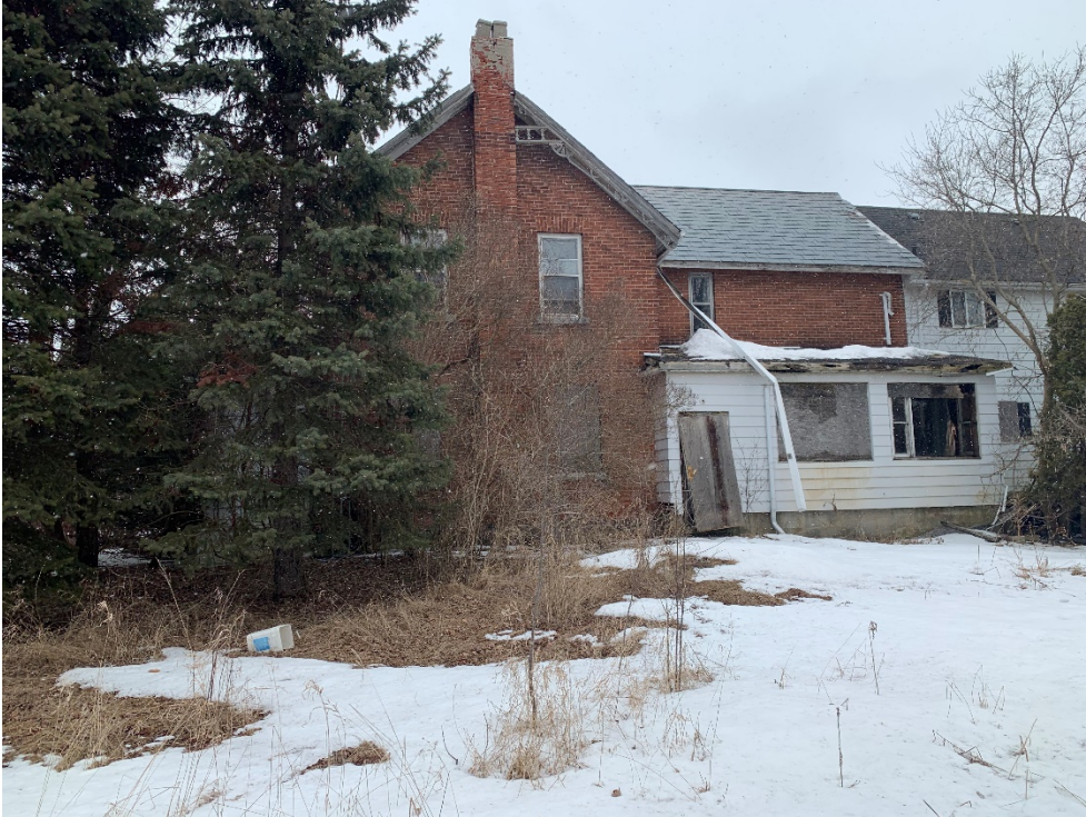
Figure 16: South elevation showing chimney, brickwork, and additions (CU 2020).
