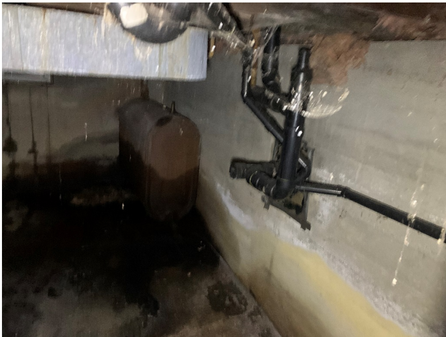
Figure 31: View of basement (CU 2020).
