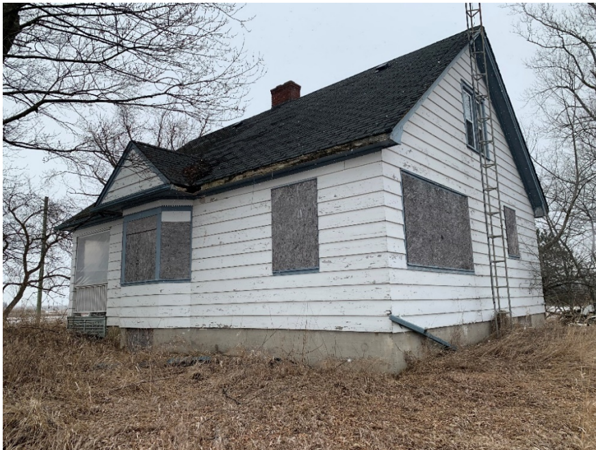
Figure 27: Front façade, cutaway porch on the left (CU 2020).
