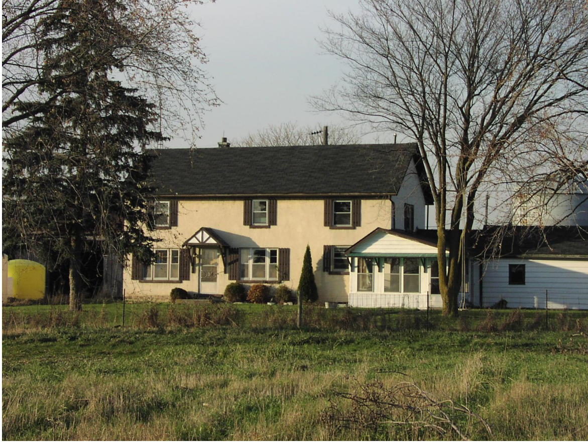
Pingle-Brown House 4638 Major Mackenzie Drive
