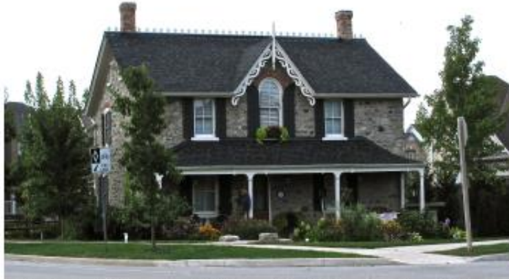
Heritage structure located on a corner lot, with strong relationship between front door and the street
