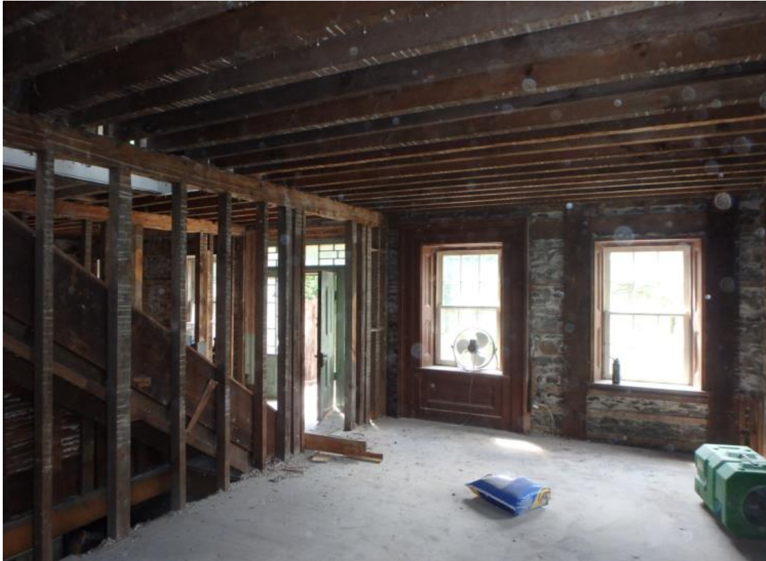
Interior – all walls back to studs
