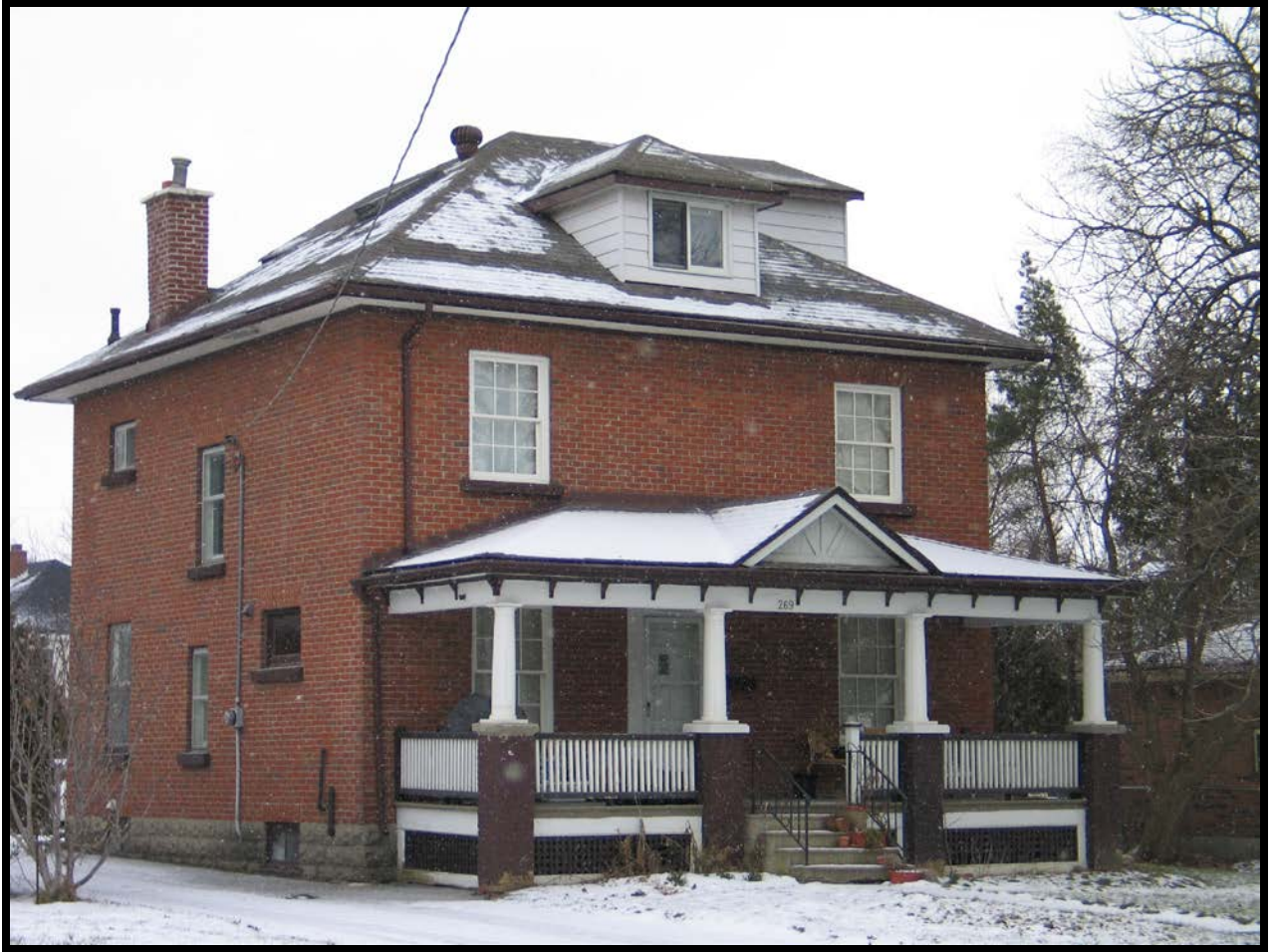
Figure 2- Photograph of existing heritage dwelling
