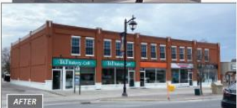
Remodeling of the exterior at 27-37 Main St. N Markham
