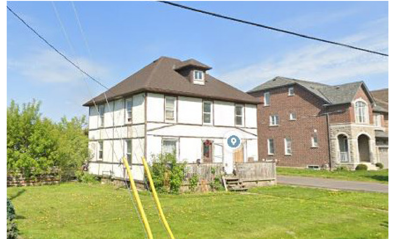
10768 Victoria Square Blvd
