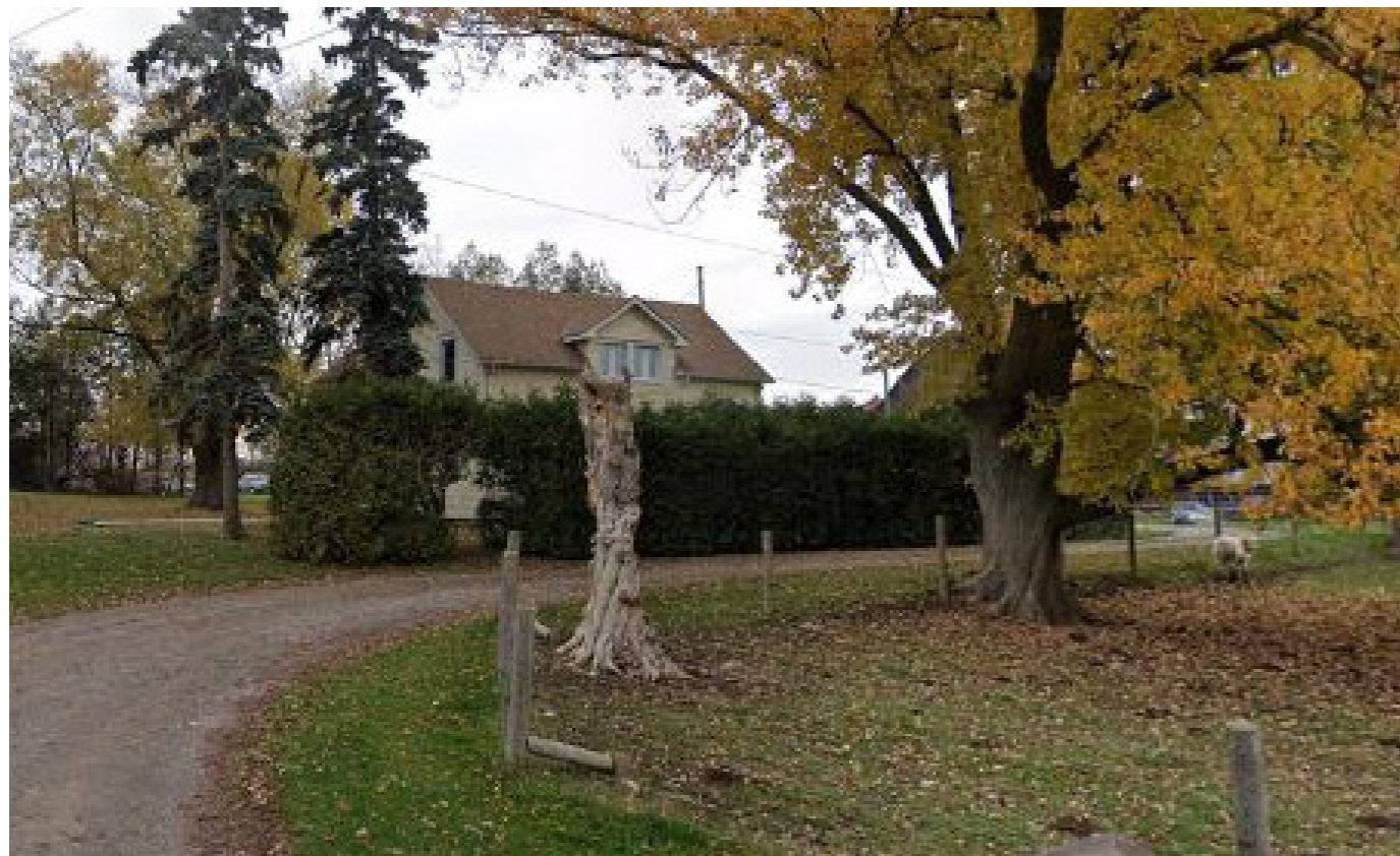
11274 Reesor Road (Federal)
