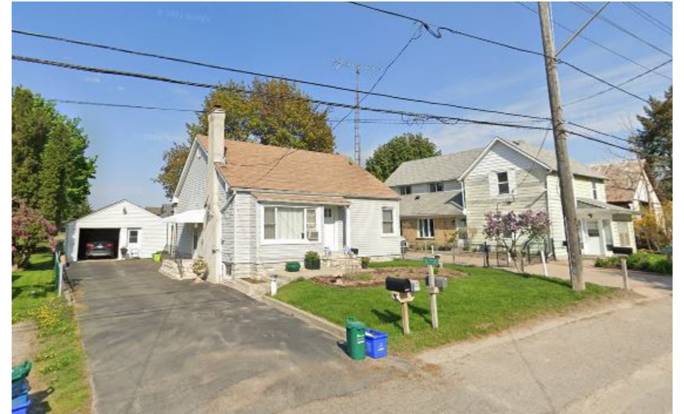
10758 Victoria Square Blvd
