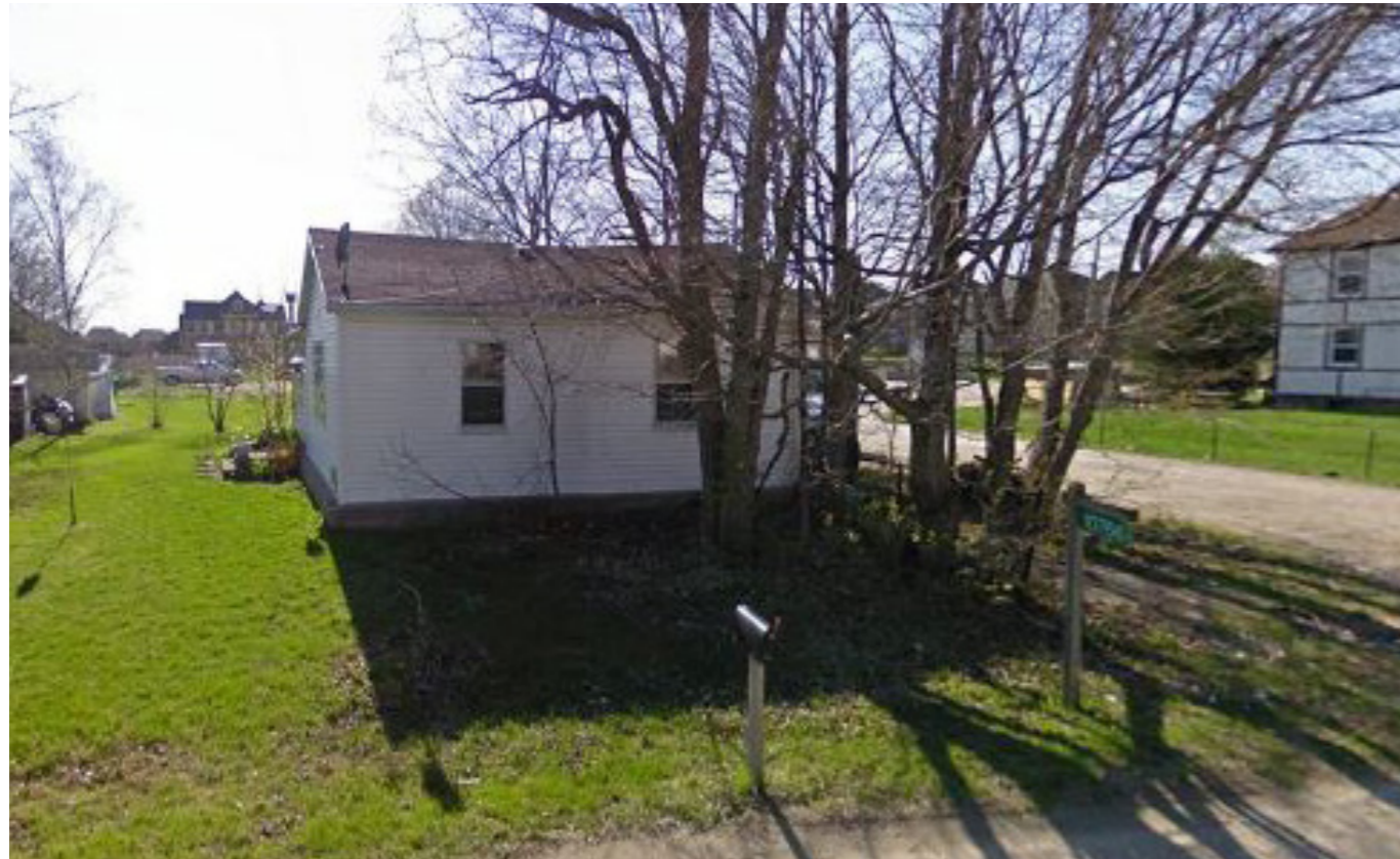
10766 Victoria Square Blvd
