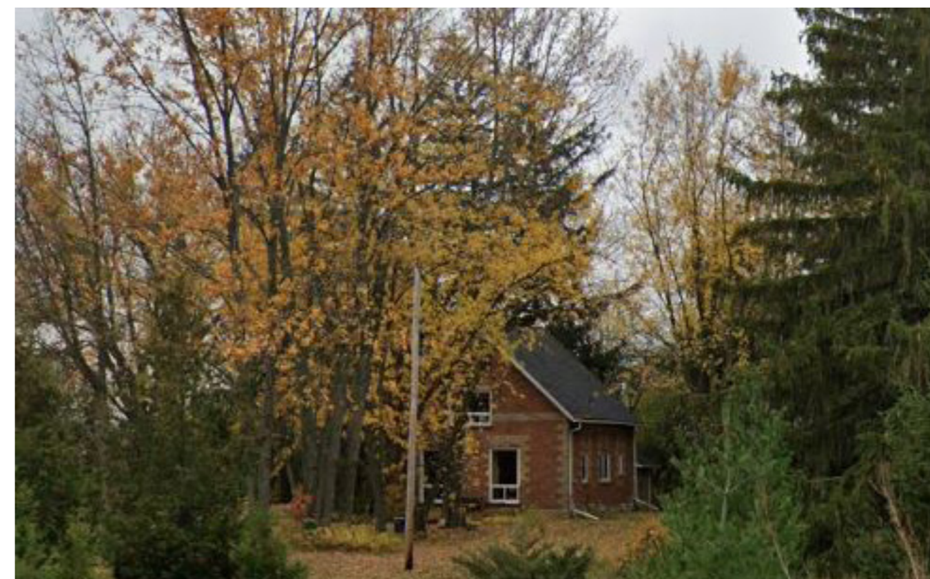
10888 Reesor Road (Federal)
