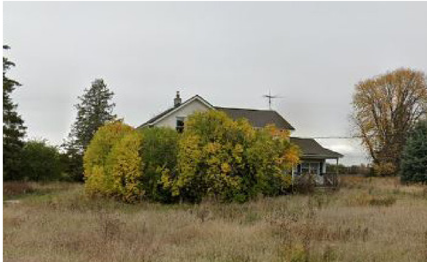
7672 Elgin Mills Road (Federal)
