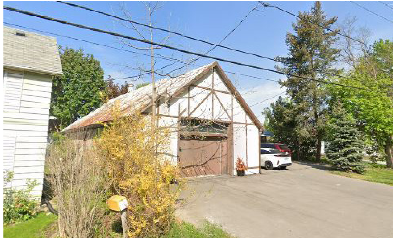
10762 Victoria Square Blvd
