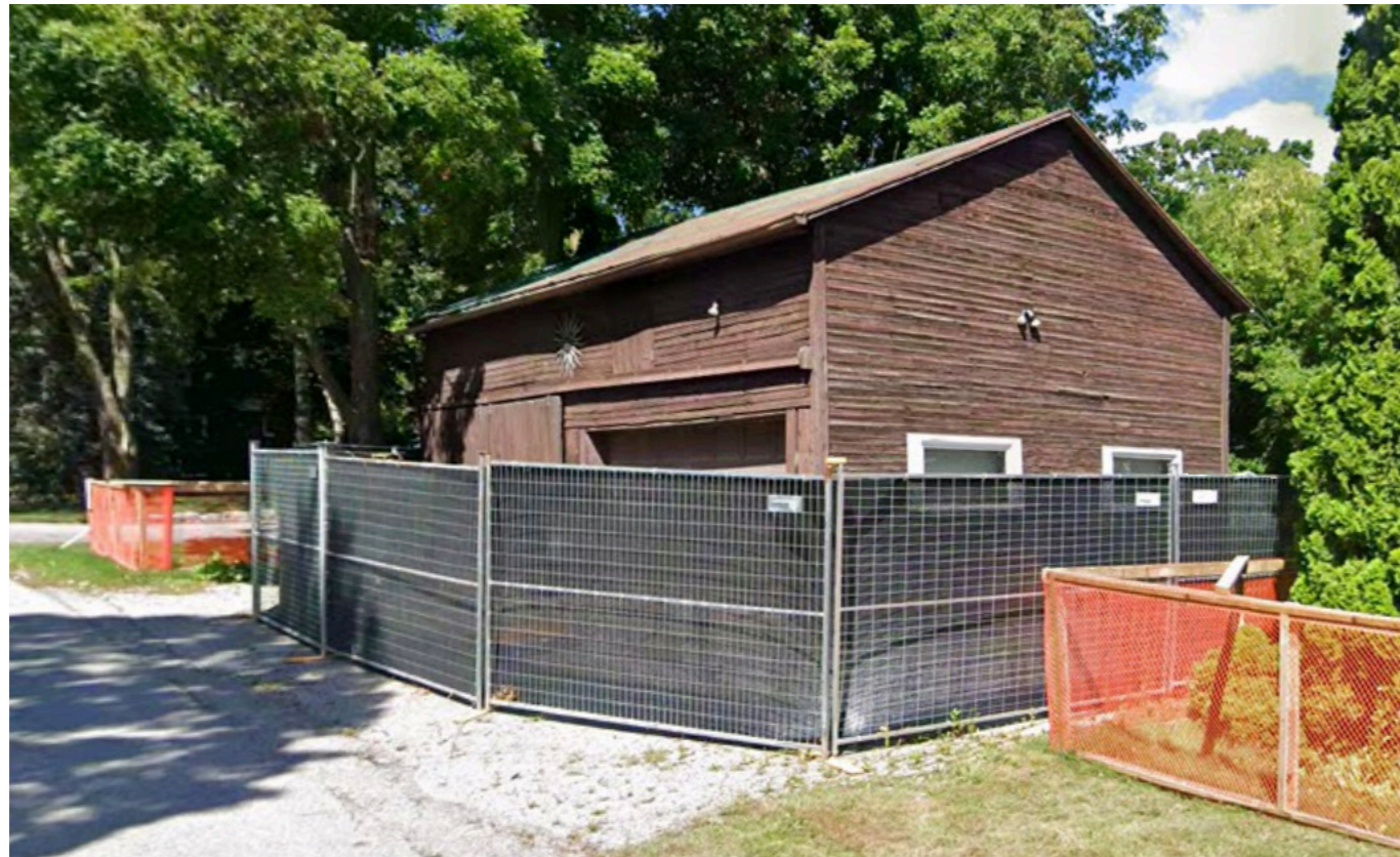
11 Victoria Street (Demolition Secured)
