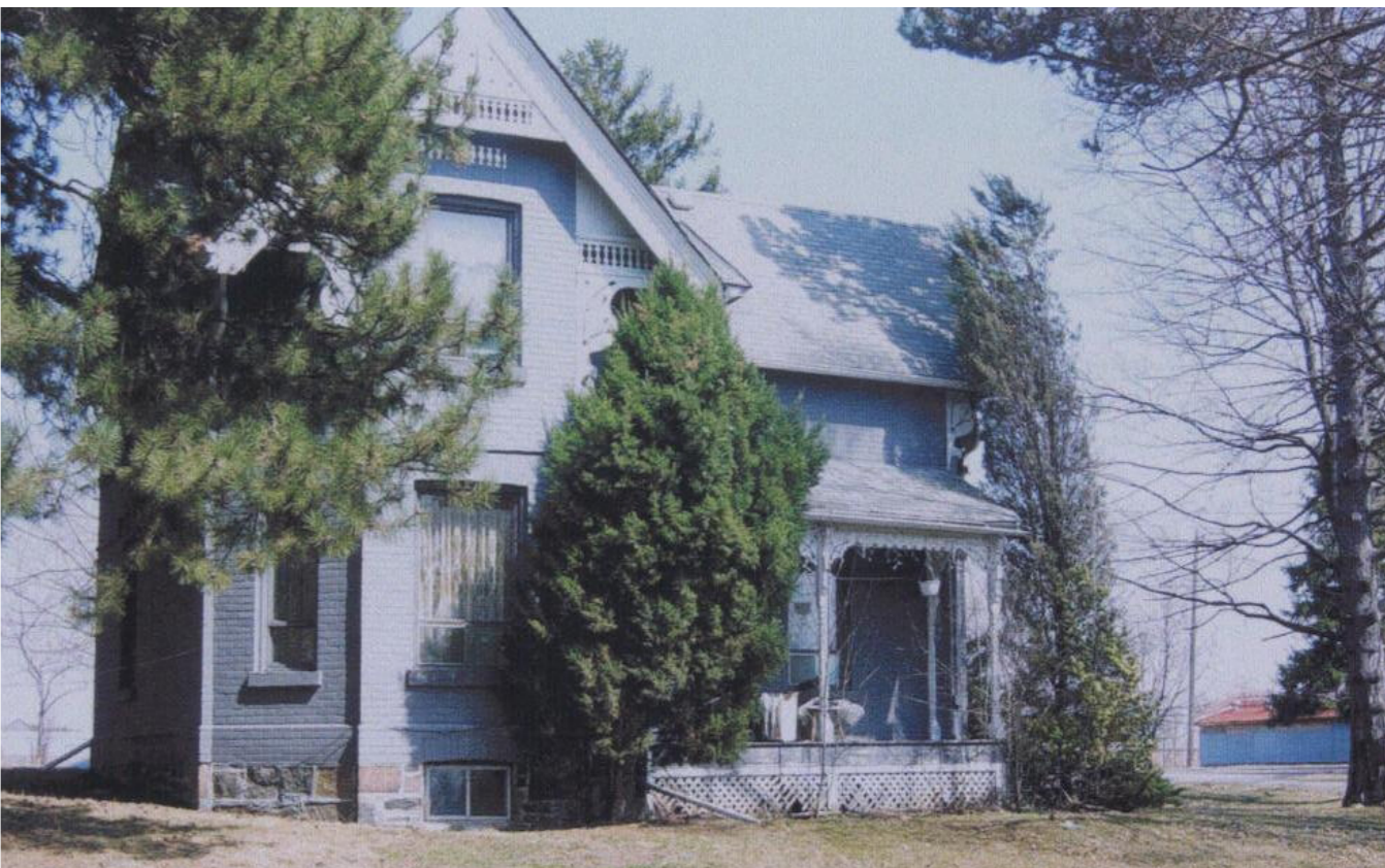
7833 Reesor Road (Federal)
