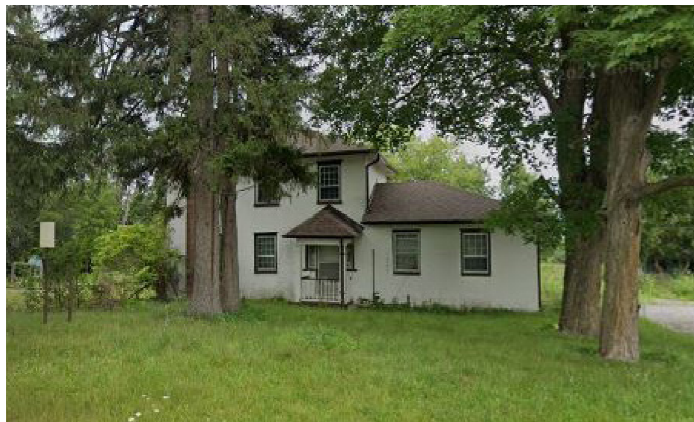
7939 Reesor Road (Federal)
