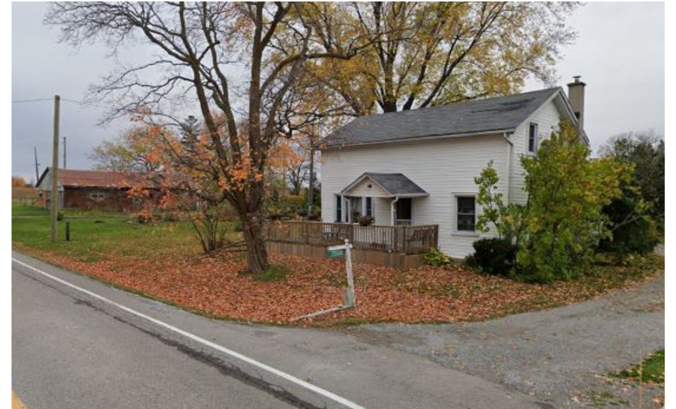
7528 Elgin Mills Road (Federal)
