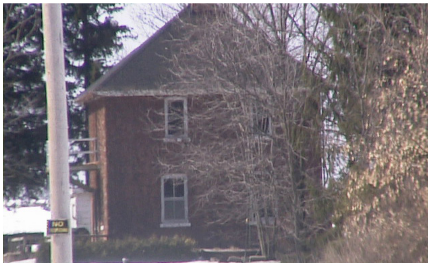
7560 11th Concession Road (Federal)
