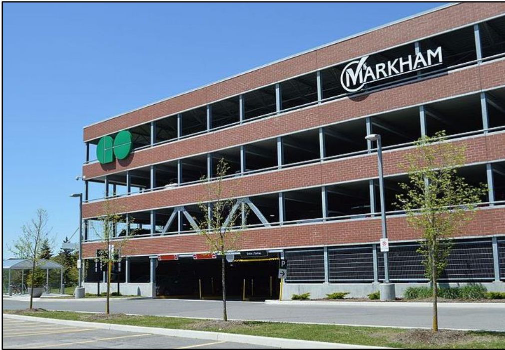
Exhibit 6-6 Prefabricated Steel Beam Parking Garage - Centennial GO Station, Markham
