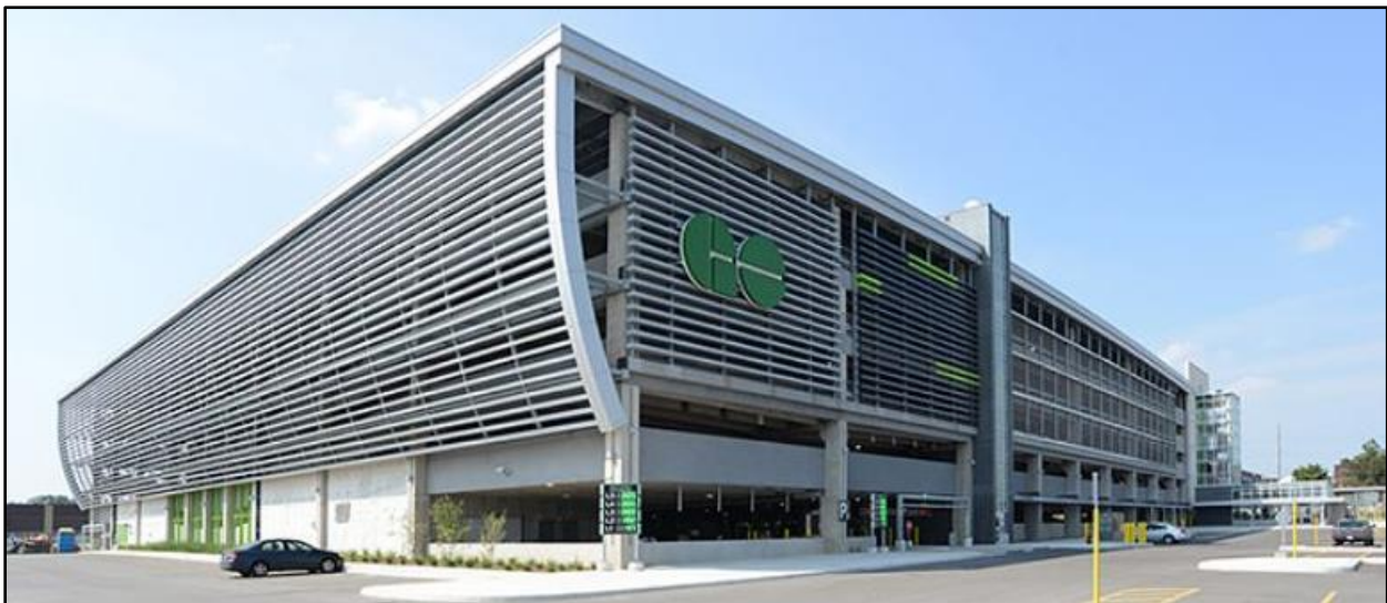
Exhibit 6-7 Precast Concrete Parking Garage - Clarkson GO Station, Mississauga
