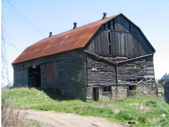
Barn at 10484 Ninth Line (Source: City of Markham)
