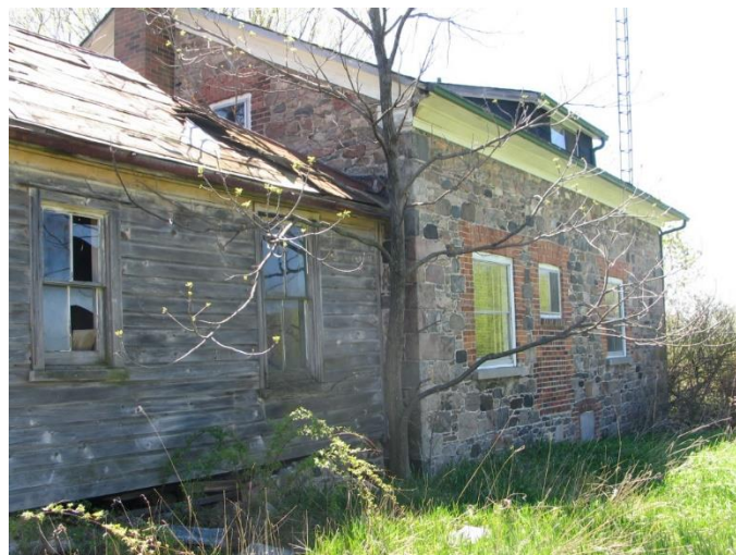
Rear view of 100484 Ninth Line (Source: City of Markham)
