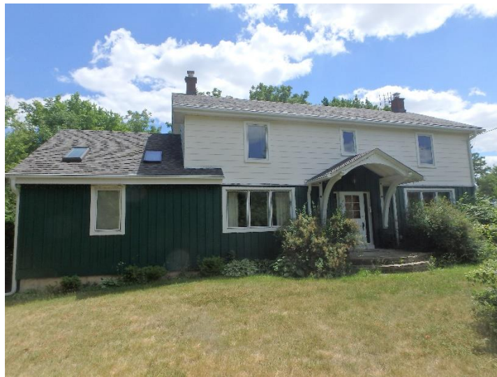
7635 Highway 7 – Front (north) elevation (Source: City of Markham)
