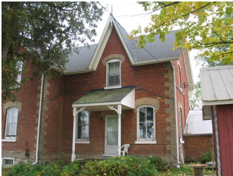
North side showing rear wing, 10224 Highway 48
