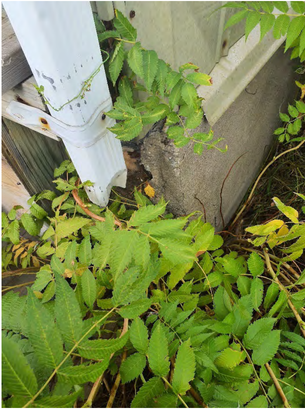
Photos 10-11- (left) Detailed view of the concealment of the original foundation clad currently in Portland Cement; (right) Detailed View of front porch/ veranda with contemporary building materials (MHBC, 2023).
