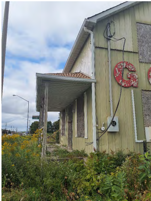
Photos 10-11- (left) Detailed view of the concealment of the original foundation clad currently in Portland Cement; (right) Detailed View of front porch/ veranda with contemporary building materials (MHBC, 2023).
