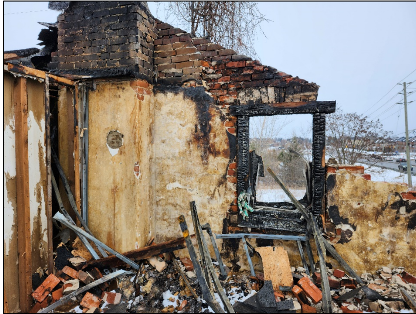
Photograph 5: Partially collapsed east gable wall
