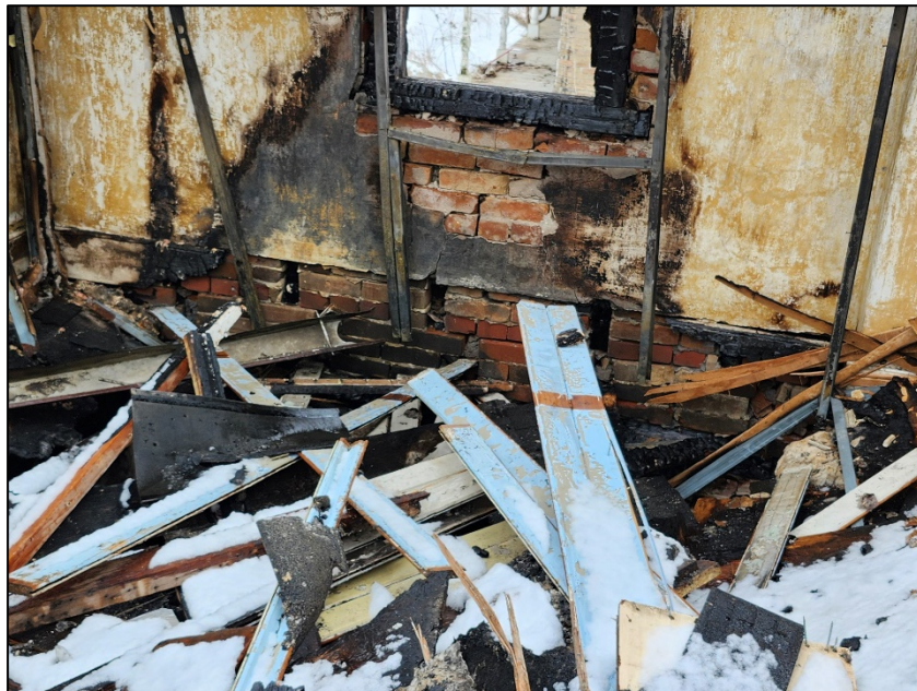
Photograph 8: Collapsed second level floor
