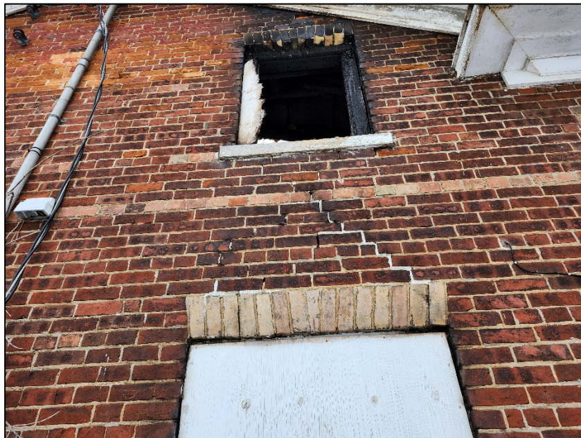
Photograph 6: Deteriorated masonry on the west gable wall
