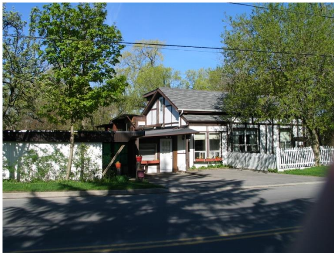
Street view of 7726 Ninth Line showing garage and link.
