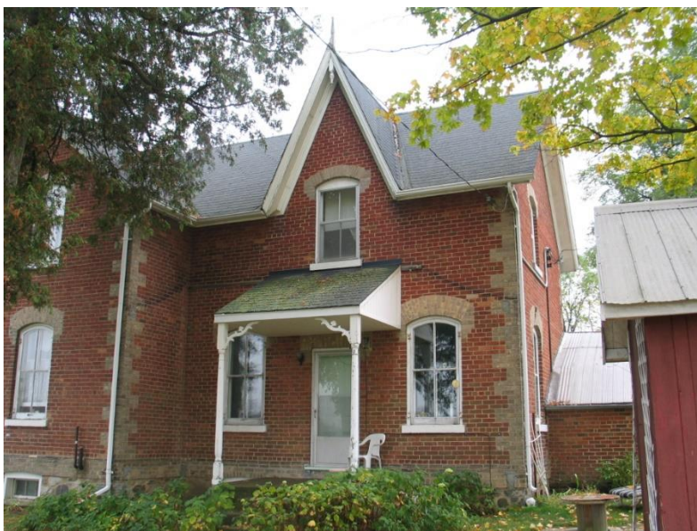
North side showing rear wing, 10224 Highway 48
