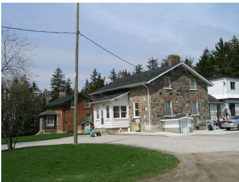
10535 and 10537 McCowan Road, showing the relationship between the two dwellings. Note the exterior cellar entrances.
