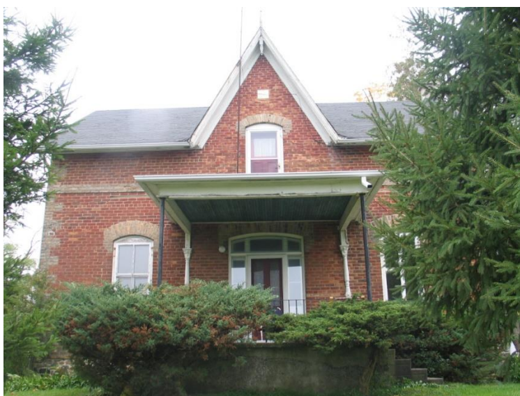
Detail of East (Front) 10224 Highway 48
