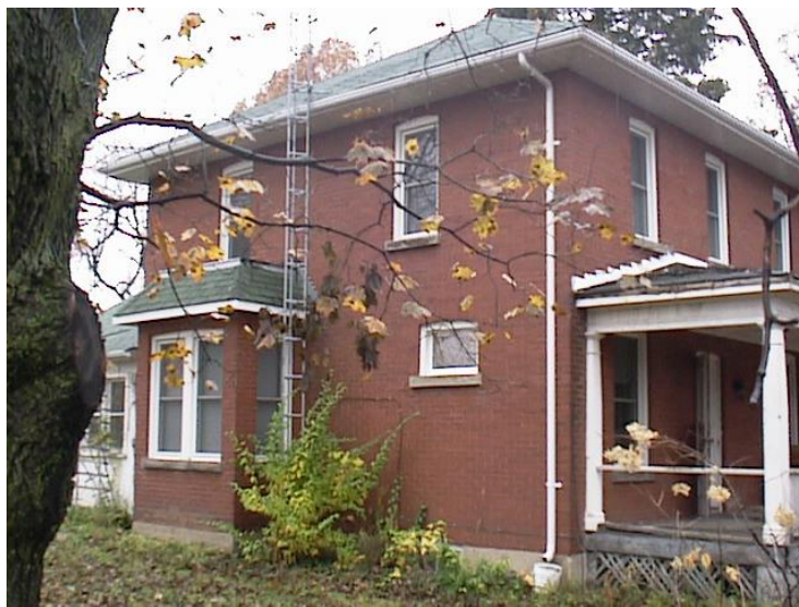
10388 Highway 48. View of south side showing box bay window.
