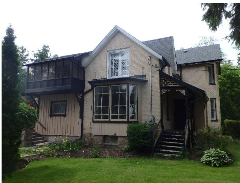
South side view of 7530 Ninth Line showing veranda detailing, south bay window and rear addition.
