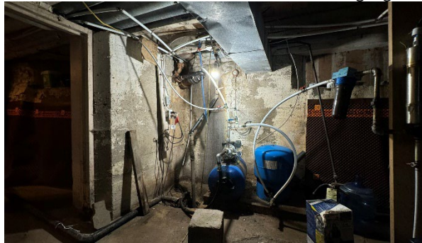
Retrofit HVAC Fixtures & Concrete Parging
