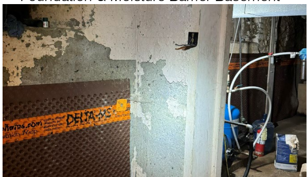
Foundation & Moisture Barrier Basement
