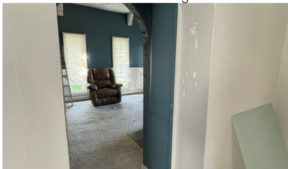
Wall Thickness Between Original & Addition
