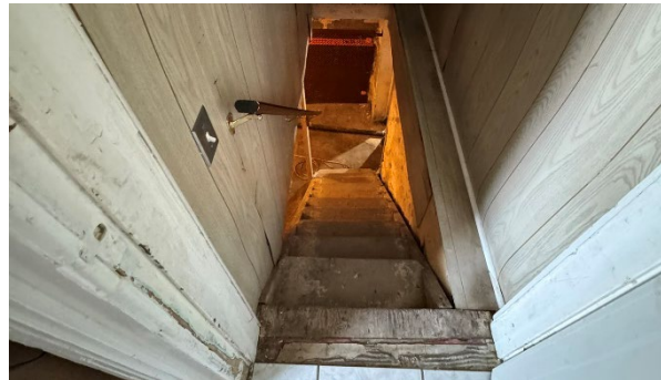
Staircase to Basement
