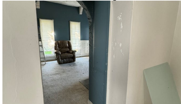
Wall Thickness Between Original & Addition
