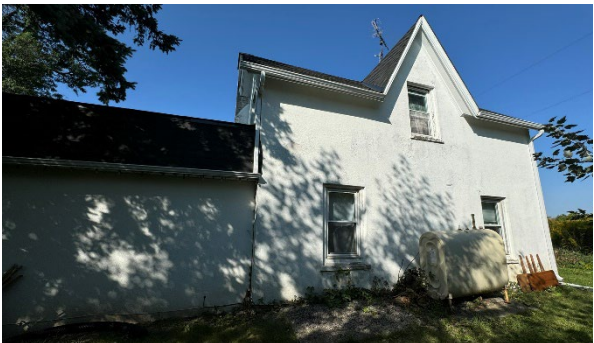
Full Extent Of East (Original Front) Façade Showing Addition & Original Sections
