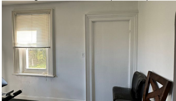
Original Front Entrance (East Side)
