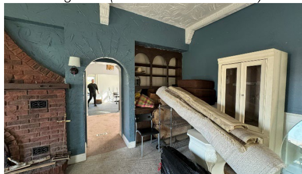
Living Area (Addition on South Side)
