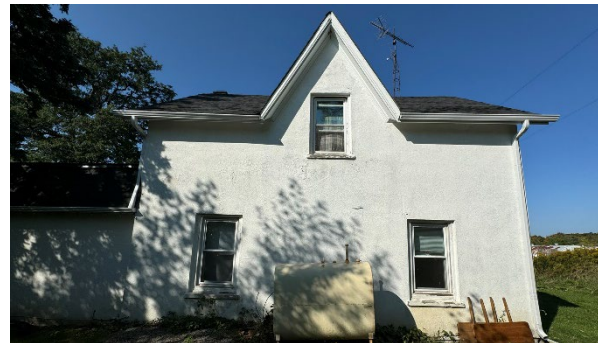
Original Section Of Farmhouse & Original East (Front) Façade With Bricked Over Front Entrance and Peaked Dormer
