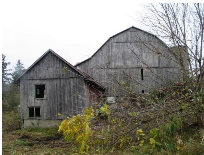
Raymer Farm barn complex, north of the farmhouse (demolished).
