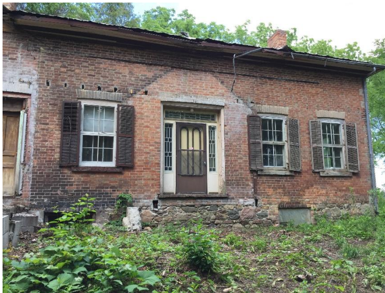
Front view taken in 2021 with doddy house removed. Note the door on the left, originally a window.
