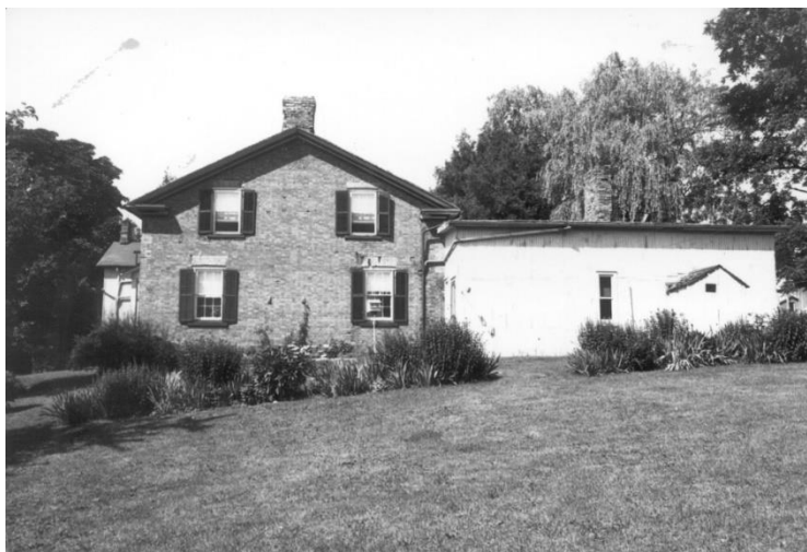
East side view from 1981 showing rear addition.
