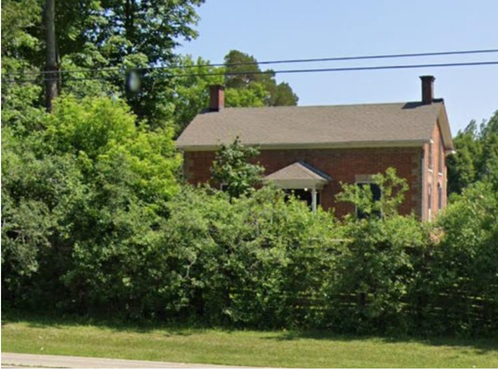
The north (primary) elevation of the heritage resource as seen in June 2023 (Source: Google Earth)
