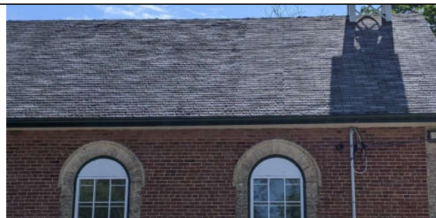
Photo 2: Degranulation and curling of shingles at roof.
