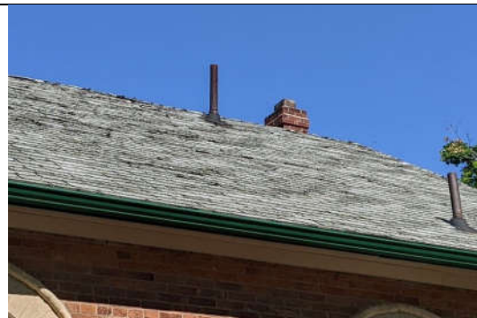
Photo 2: Degranulation and curling of shingles at roof.
