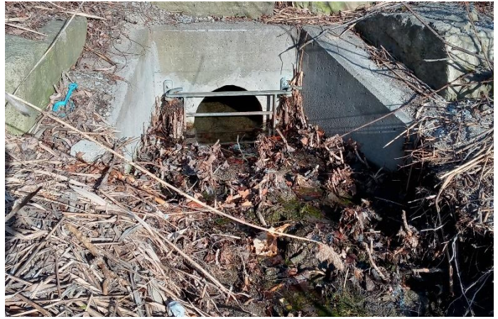
East Pond Mid-Splitter After Cleaning (April 2022)
