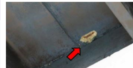
Image 2 – Concrete spall at underside of precast double-tee above swimming pool area
