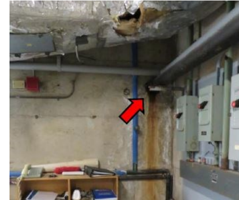
Image 3 – leak at pipe seal near circuit breakers
