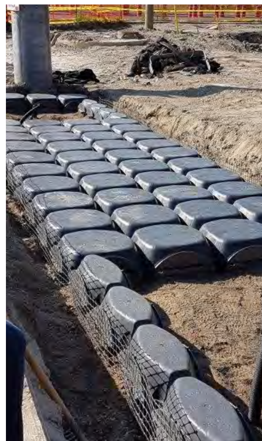
Installation of a soil cell system
