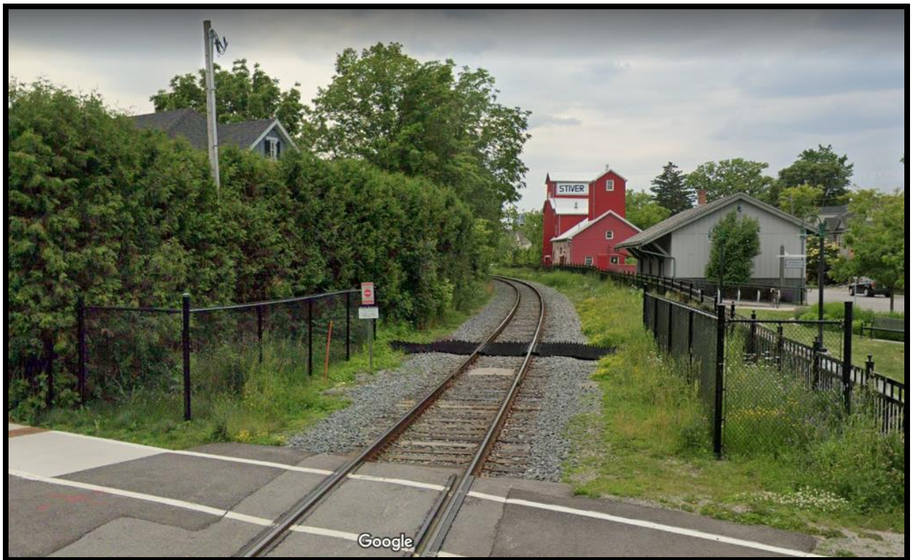
Figure 5- Photograph of existing chain link fence around railway tracks
