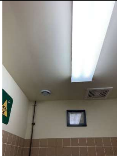
Washroom ceiling drywall
