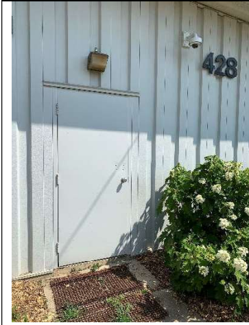
Painted metal door with frame
