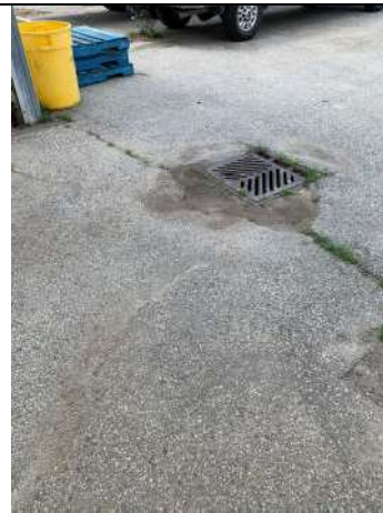
Central greenhouse asphalt
