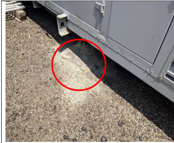
Photo 1: Roof repair to address leak.
