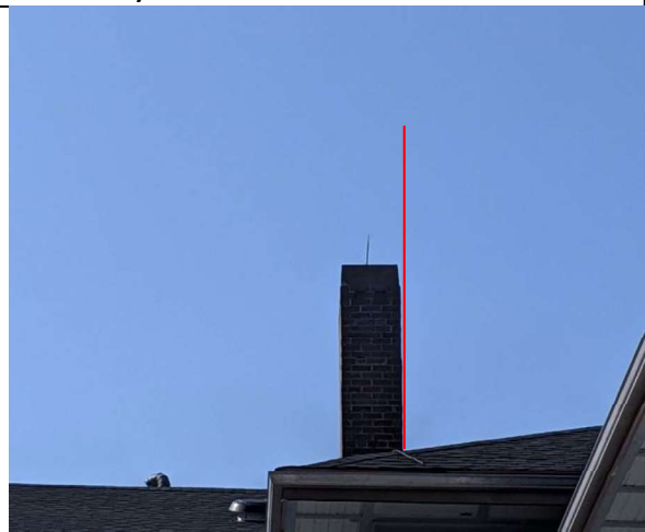
Photo 4: Smaller chimney is not quite vertical.
