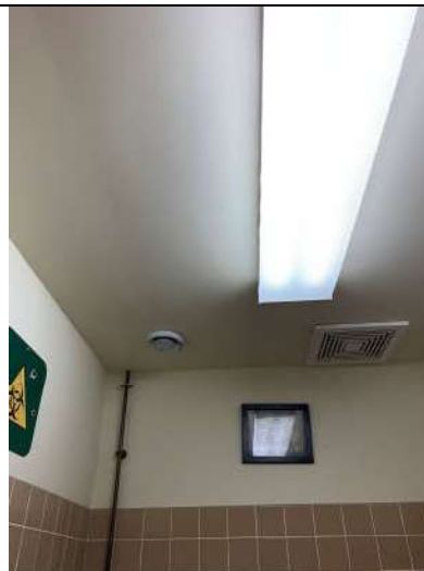
Washroom ceiling drywall
