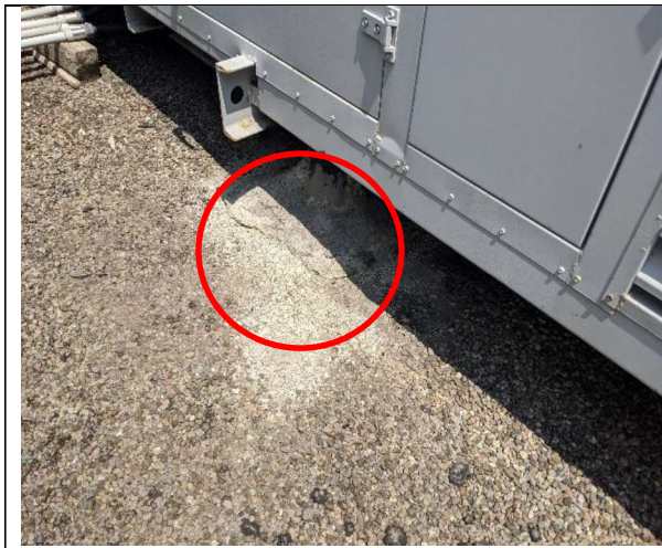
Photo 1: Roof repair to address leak.
