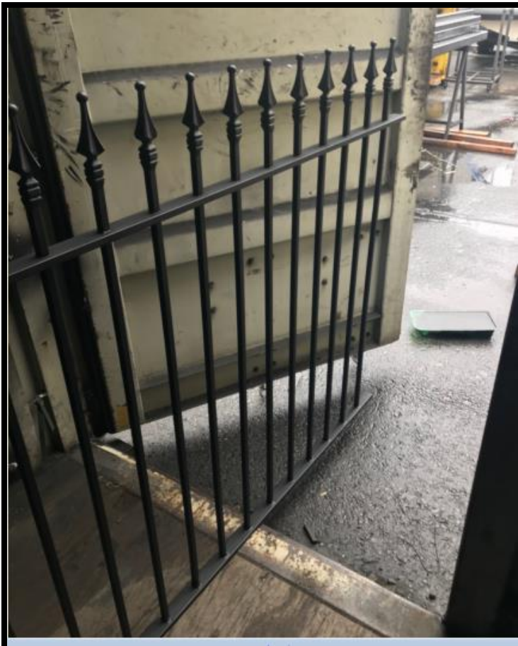
Detail of proposed replacement wrought iron fence with tubular steel posts
