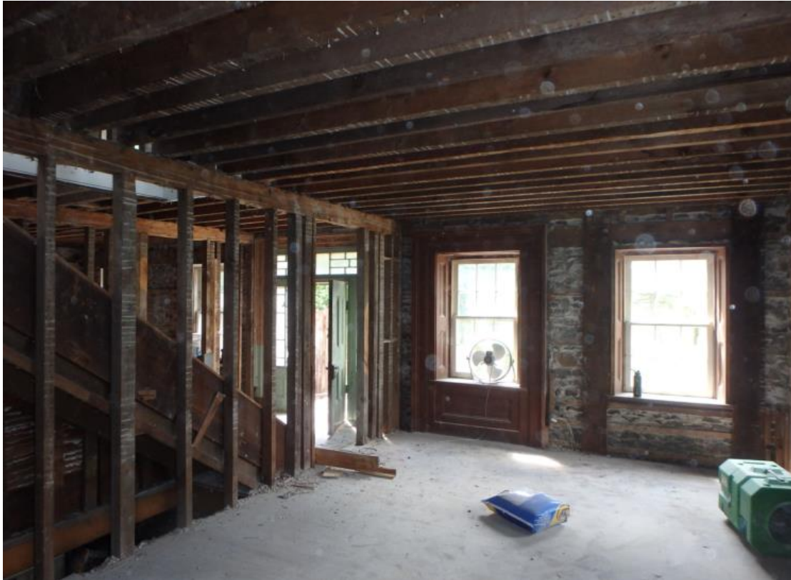
Interior – all walls back to studs
