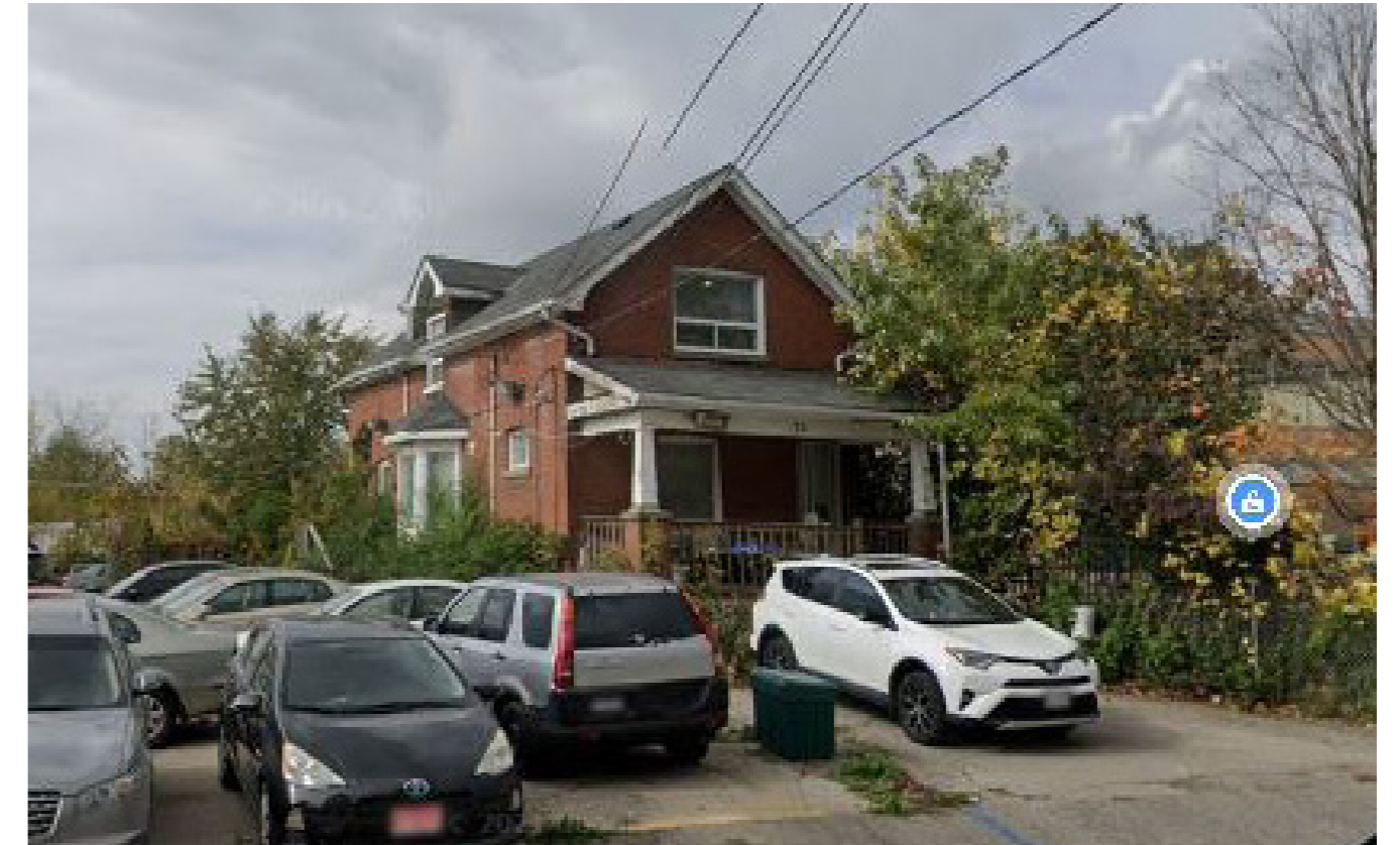
64 Old Kennedy Road (Demolition Secured)
