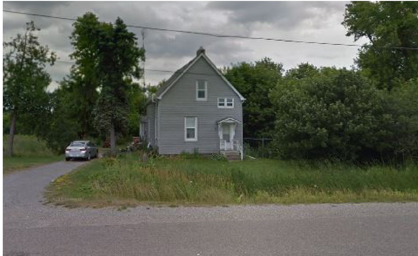
165 Locust Hill Lane (Federal)
