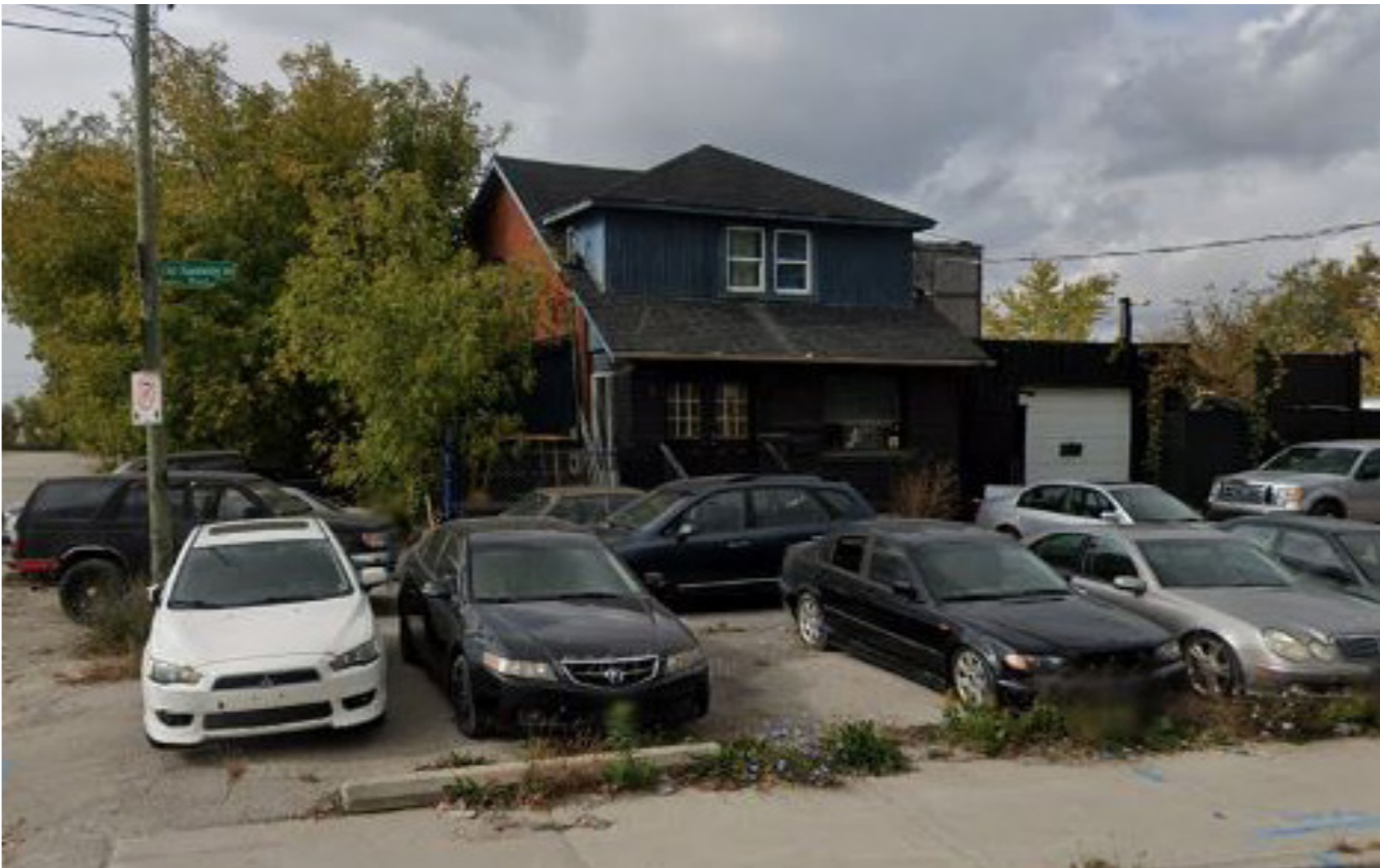
58 Old Kennedy Road (Demolition Secured)
