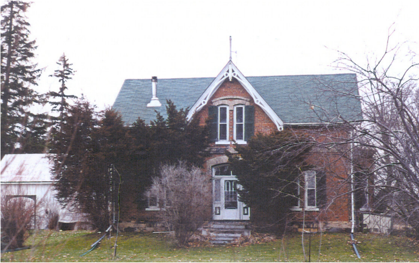
20 Locust Lane (Federal)
