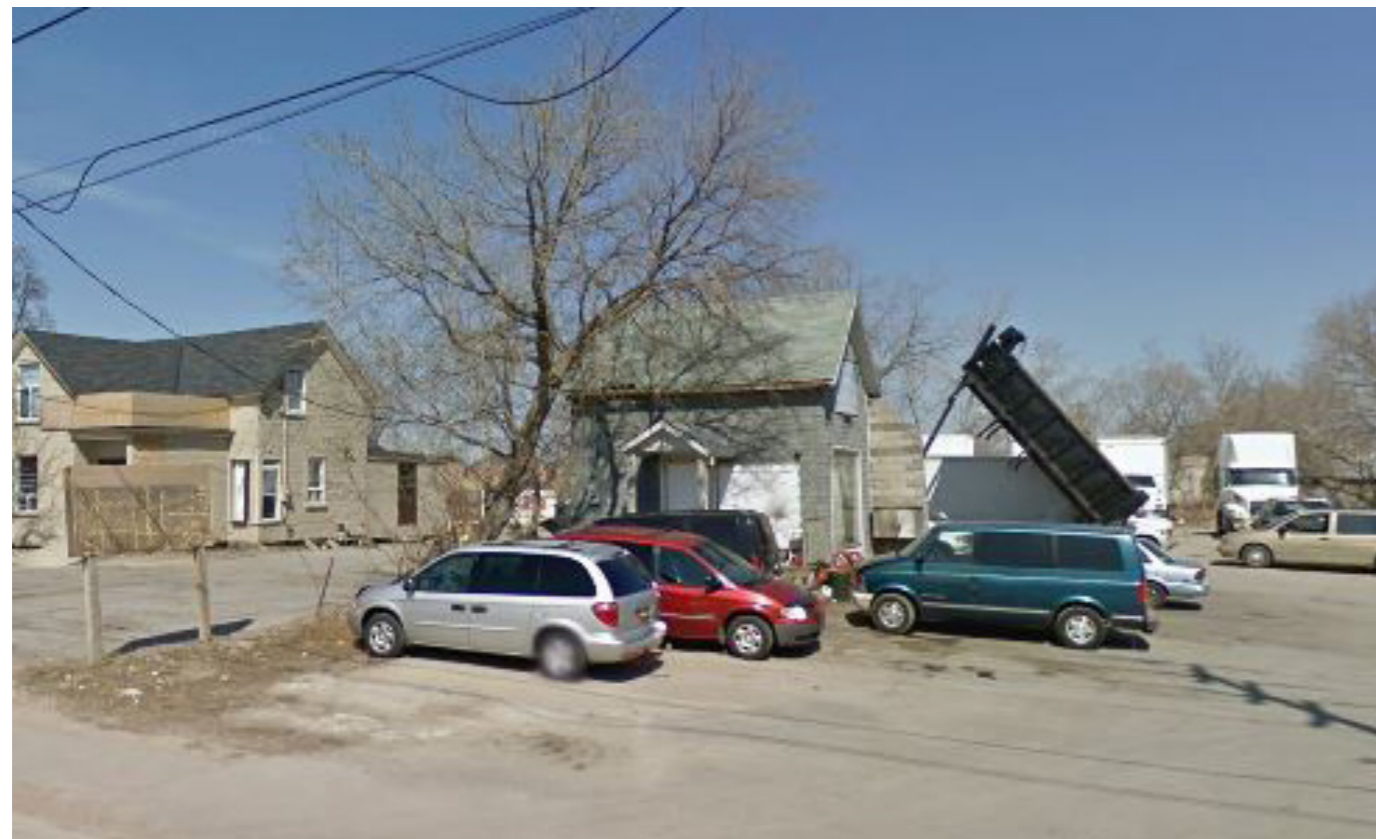
51 Old Kennedy Road (Demolition Secured)
