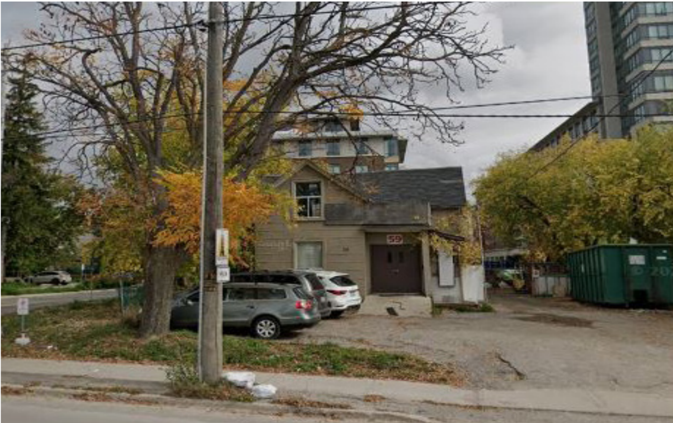
59 Old Kennedy Road (Demolition Secured)
