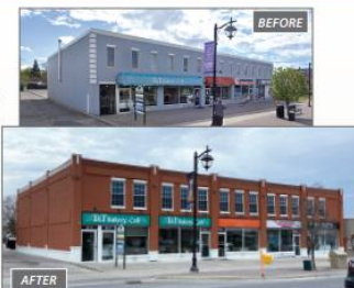
Remodeling of the exterior at 27-37 Main St. N Markham
