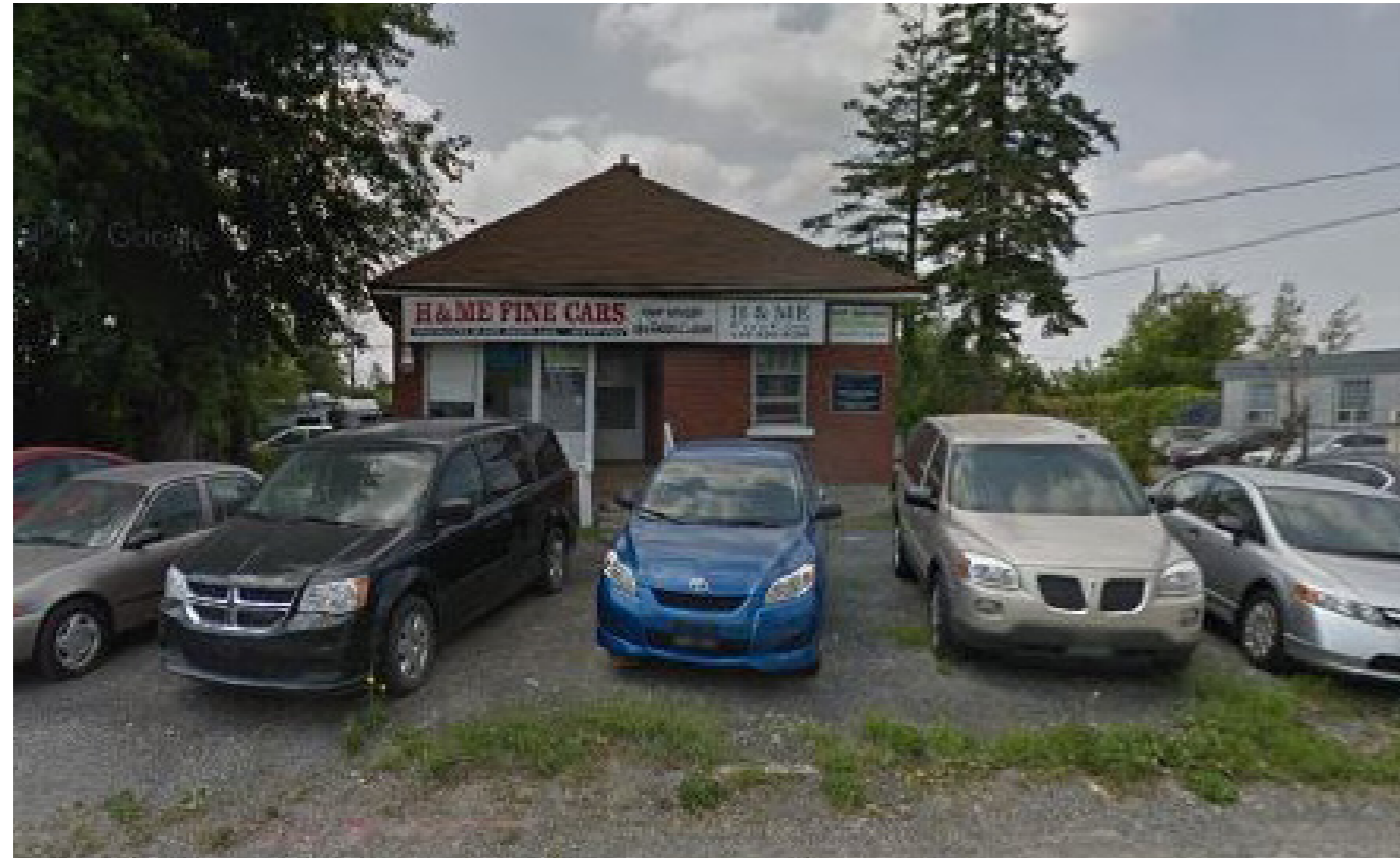
30 Old Kennedy Road (Demolition Secured)
