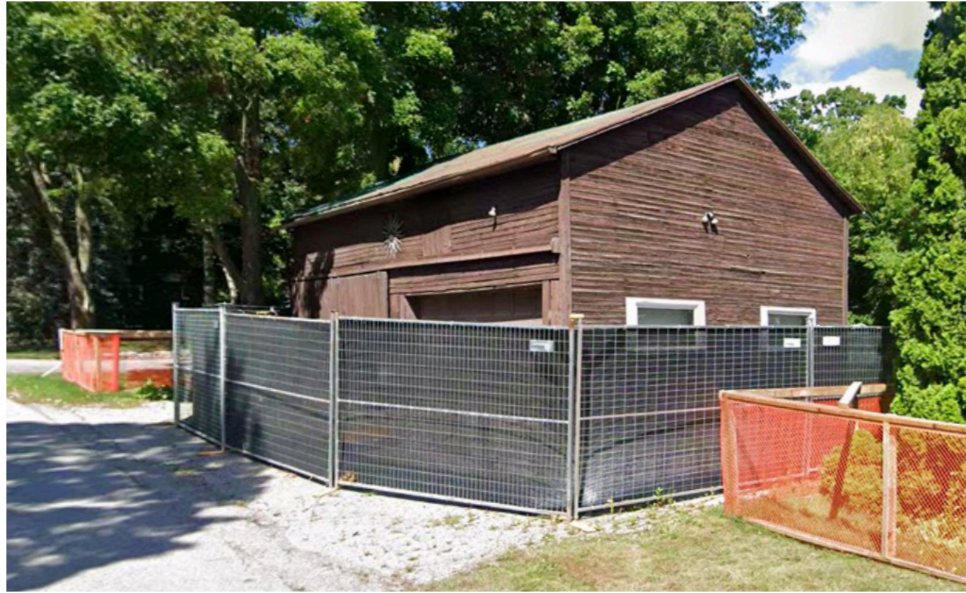
11 Victoria Street (Demolition Secured)
