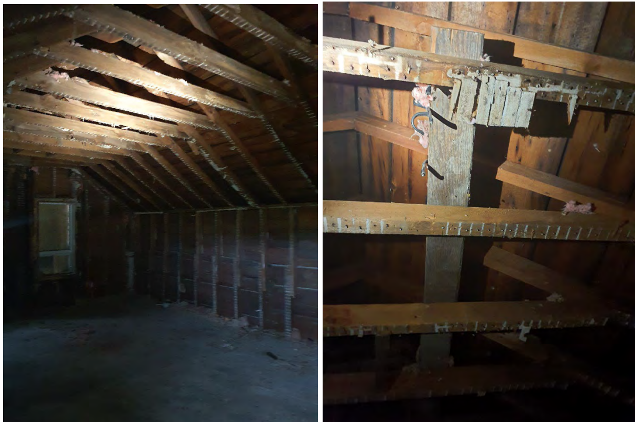
Photos 14-15- (left) View of current roof structure which has been replaced predominately with contemporary materials; (right) Detailed view of existing roof structure and removal of former lathe and plaster (MHBC, 2023).
