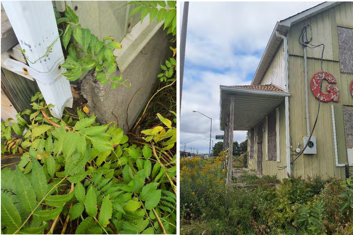
Photos 10-11- (left) Detailed view of the concealment of the original foundation clad currently in Portland Cement; (right) Detailed View of front porch/ veranda with contemporary building materials (MHBC, 2023).
