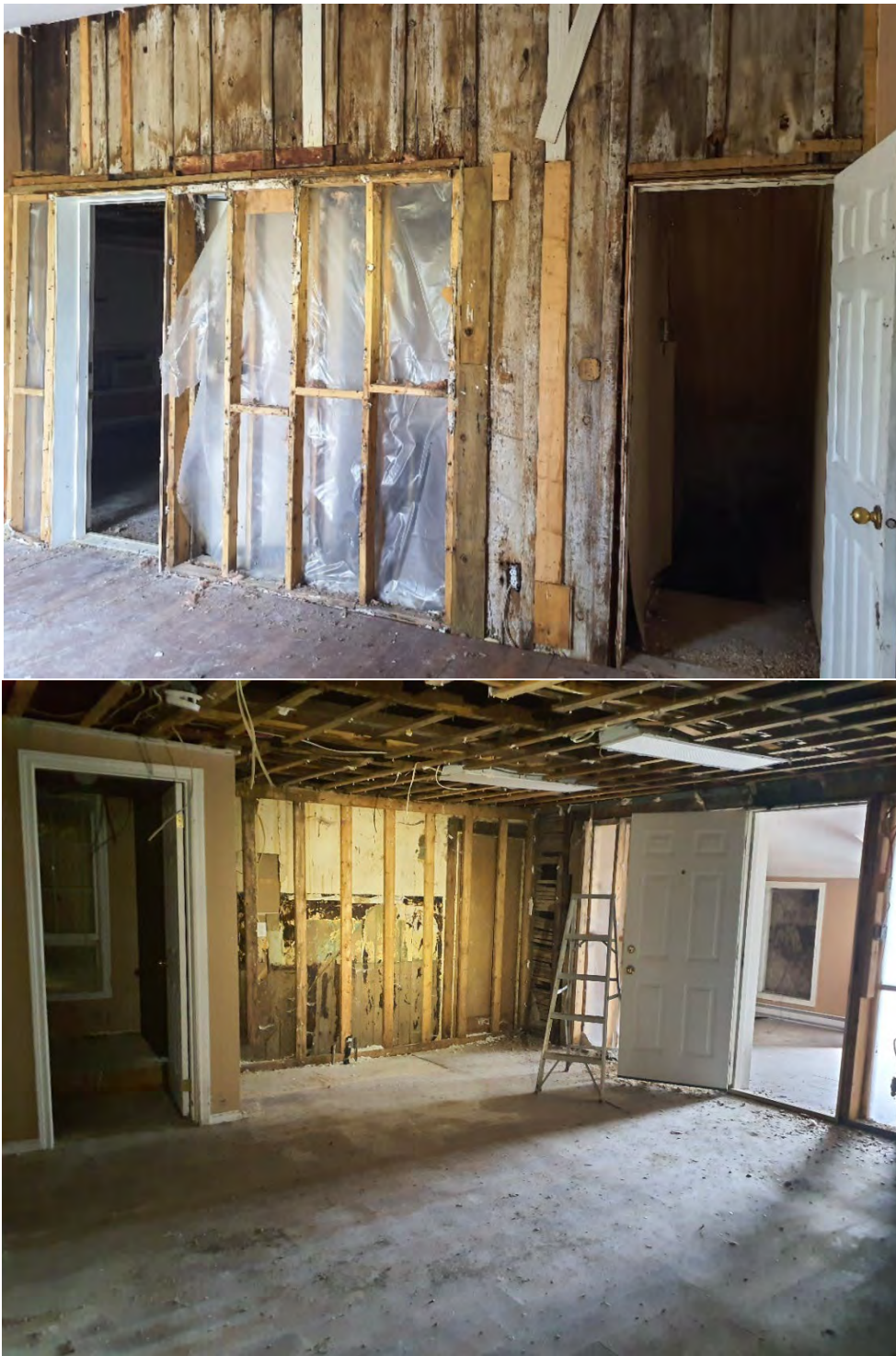
Photos 12-13- (above) View of only exposed wall (north elevation) of original building construction shown within rear addition showing significant alterations including new openings and unsympathetic replacement of materials; (below) View of the interior of the main building showing significant alterations including contemporary changes to the building structure by replacement of materials, replacement of original doors, window frames and flooring (MHBC, 2023).
