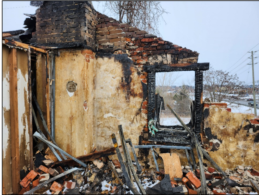
Photograph 5: Partially collapsed east gable wall
