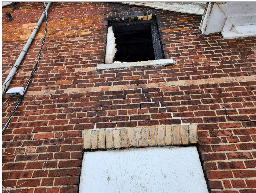
Photograph 6: Deteriorated masonry on the west gable wall
