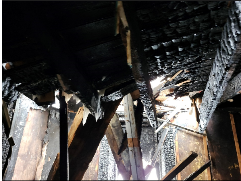
Photograph 7: Collapsed second level floor
